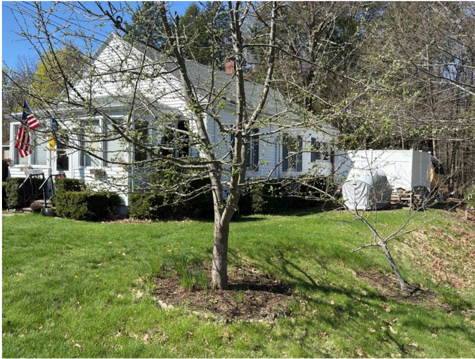
31. Southern adjoining single-family residence (408 Auburn Street)
