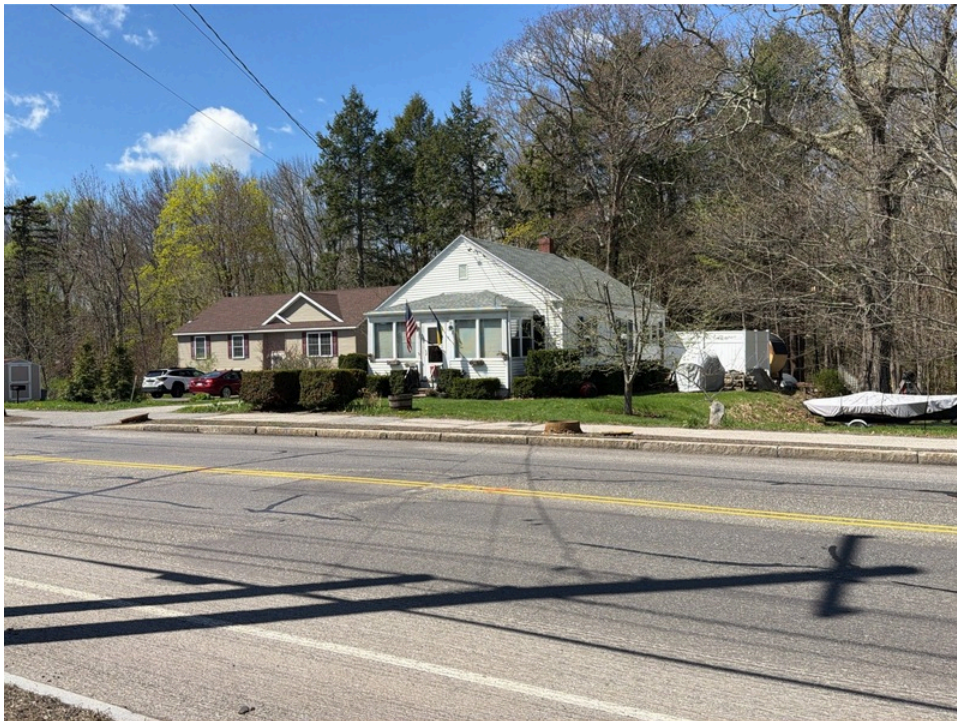
32. Southern adjoining single-family residences (372-408 Auburn Street)
