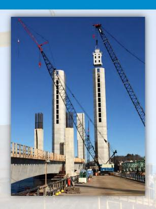
Tower precast segments have been erected
