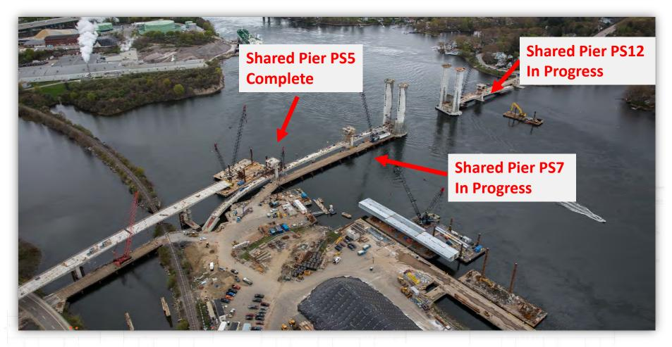
Each of the (3) shared piers are underway – segment erection has started on the PS5 cantilevers
