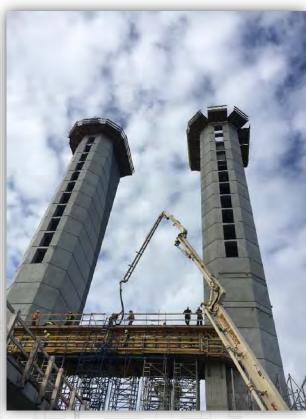
Above – Pier 9 Vehicle Approach Beam Concrete Placement
