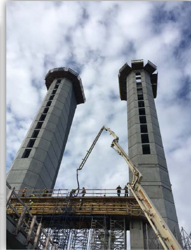
Above – Pier 9 Vehicle Approach Beam Concrete Placement
