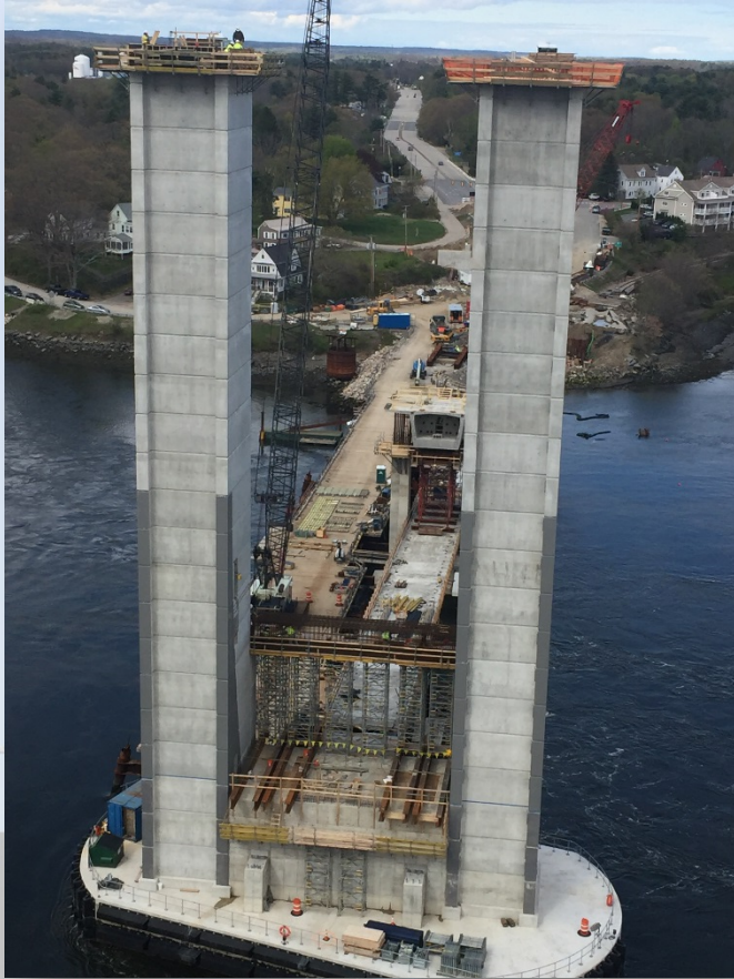
Kittery Tower & Machine Room – Vehicle beam in progress
