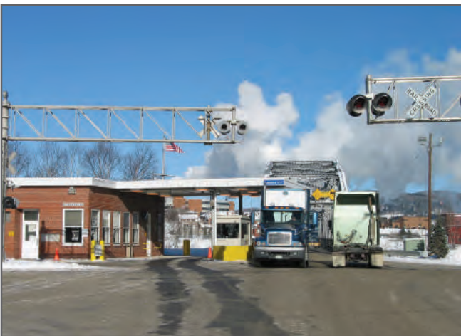
The existing LPOE main building, looking north. Photo shows the lack of an outbound inspection lane.
