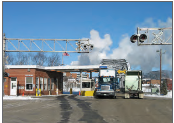
The existing LPOE main building, looking north. Photo shows the lack of an outbound inspection lane.
