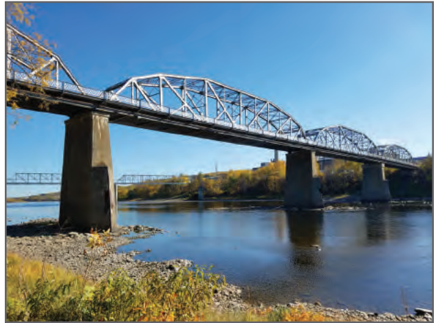
The existing International Bridge, from the bank of the Saint John River on the Edmundston Side looking southeast.
