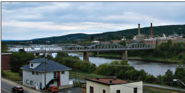
The existing International Bridge from Edmundston, looking southeast.
