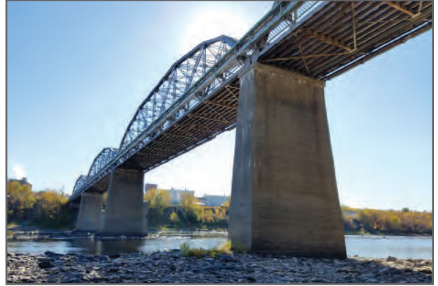
The existing International Bridge from the bank of the Saint John River on the Madawaska side looking at the substructure.
