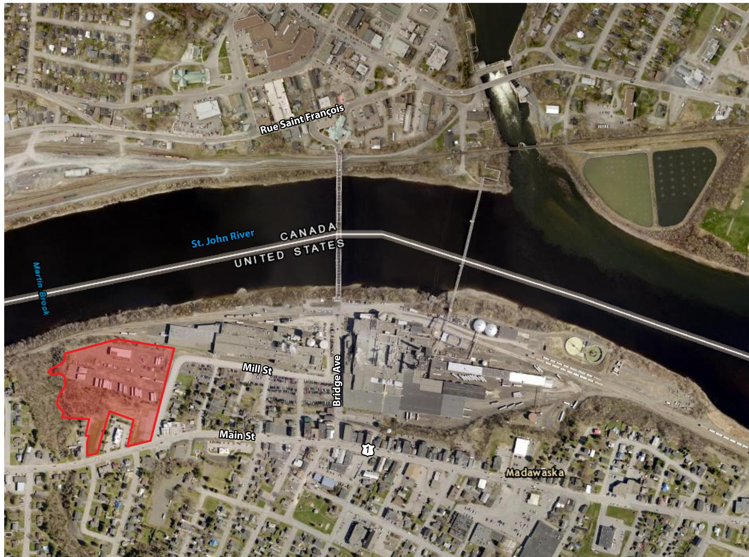
Madawaska/Edmundston International Bridge and Border Crossing
