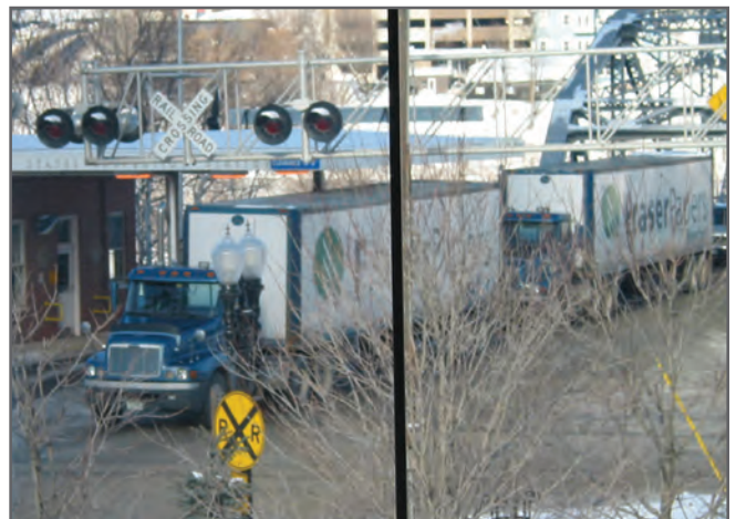
The existing LPOE, looking north. Photo shows the lack of space for an inbound traffic queue.
