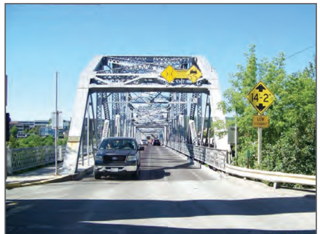
The approach to the existing International Bridge from the existing Madawaska LPOE.
