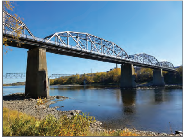
The existing International Bridge, from the bank of the Saint John River on the Edmundston Side looking southeast.
