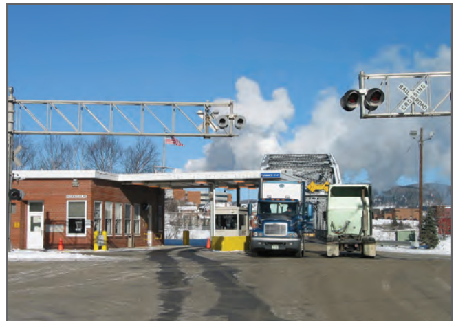
The existing LPOE main building, looking north. Photo shows the lack of an outbound inspection lane.
