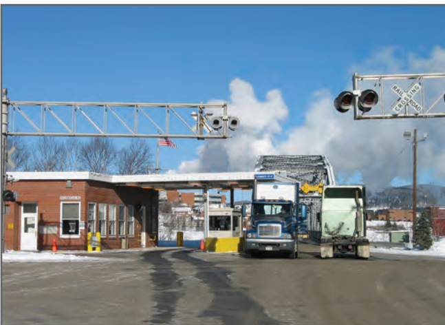
The existing LPOE main building, looking north. Photo shows the lack of an outbound inspection lane.
