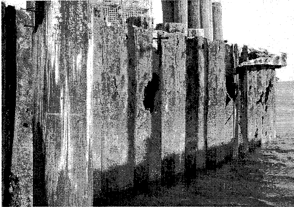
Photo # 3, South pier, Station 18 – 50, general conditions above the water line
