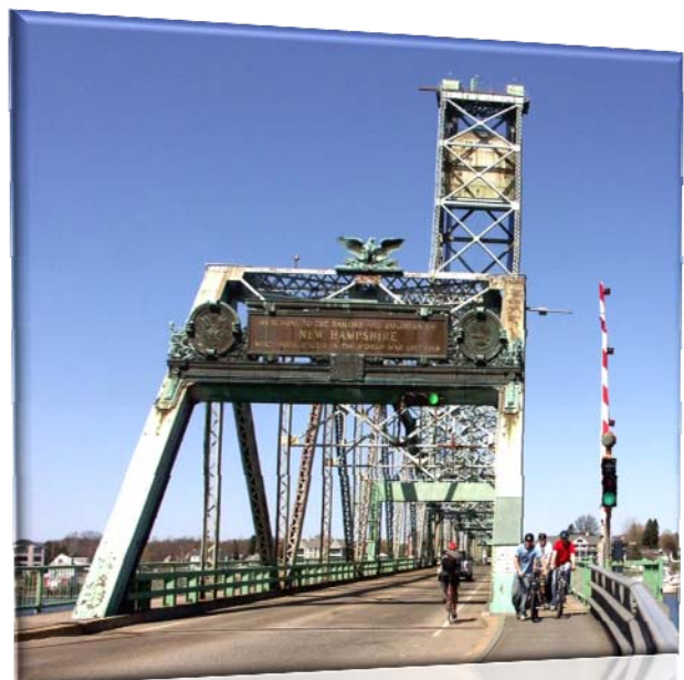
Figure 5: Memorial Bridge – Existing Conditions [Source: Steve Workman]
