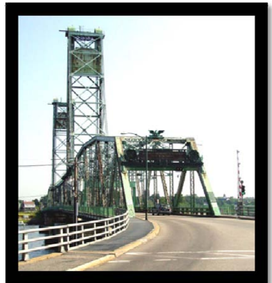
Figure 3: Memorial Bridge [Source Steve Workman]
