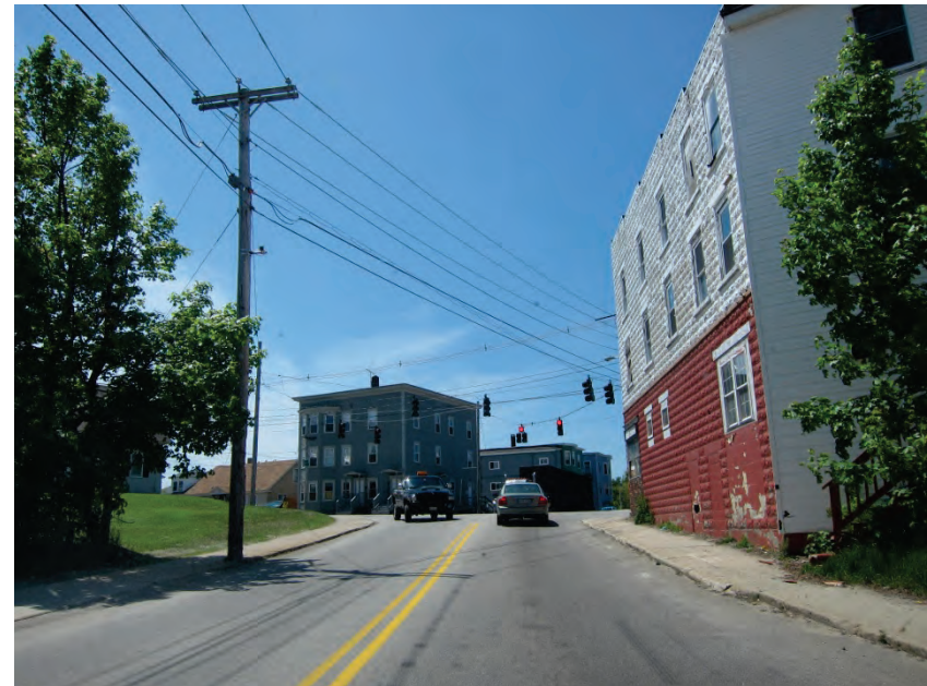
Figure 3-46: Route 202 approaching River Street (Looking West)
