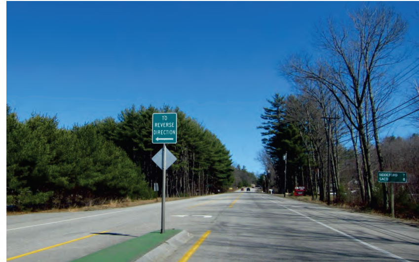
Figure 3-40: Current U-Turn on Route 111 in Lyman
