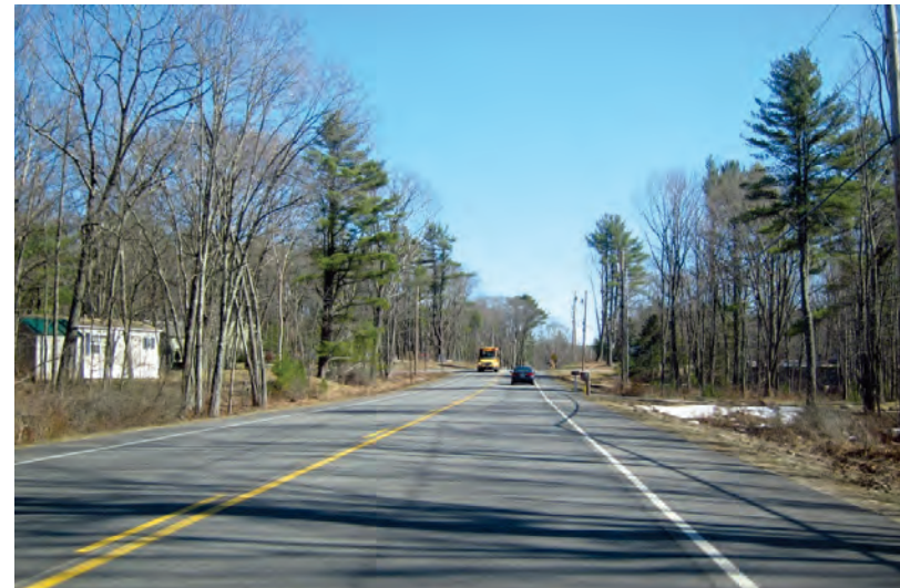
Figure 3-9: Recently Improved Section of Route 109 in Wells
