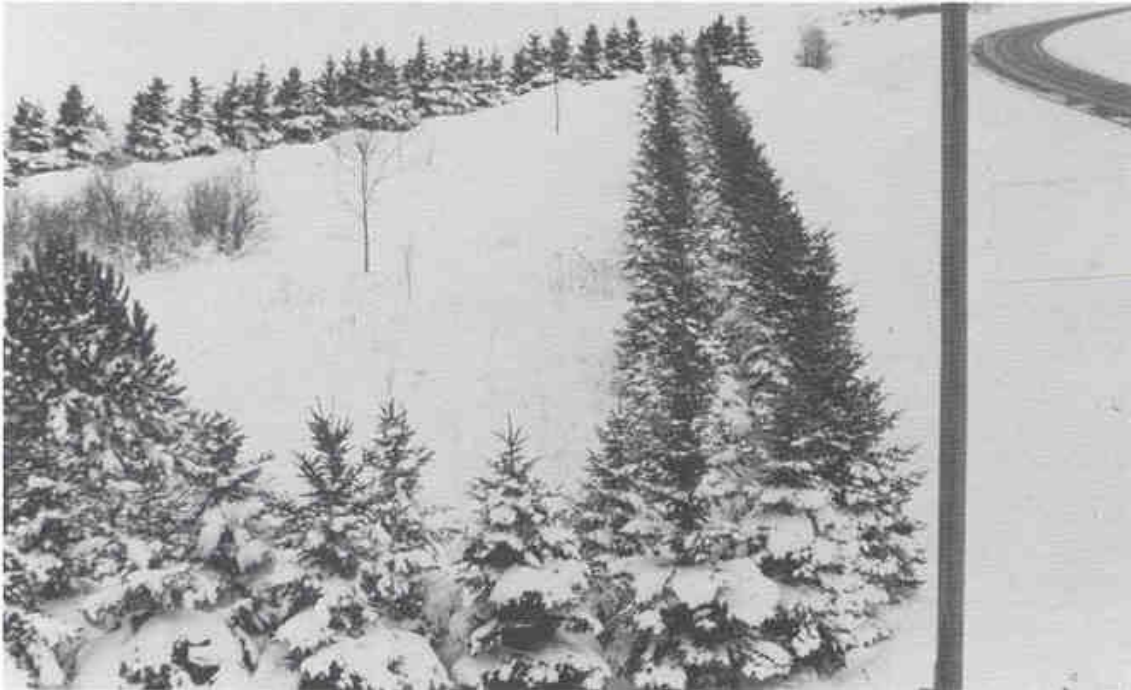
Figure 17. Living snow fences. The top photograph shows a Colorado spruce snow fence along I-35 near Owatonna, Minnesota. The bottom photograph shows the snow fence in a triangular area of a right-of-way adjacent to a separation structure across I-35. (Photographs by the Minnesota Department of Transportation.)
