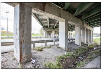
Figure 11 Under the overpass showing spalling and deterioration to the concrete.
