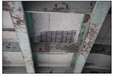
Figure 8-10 Below and above deck deterioration. Deck support structure exposed (left). Concrete bents and caps, as well as steel stringers showing the effects of weather and signs of deterioration, including spalling (center). Road surface showing signs of cracking and degrading at the point where the road meets the bridge.
