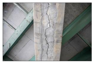
Figure 14 Cracks in concrete caps.
