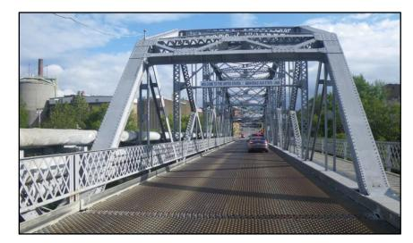
This photo, looking south towards the U.S. side of the border, shows the narrow travel lanes on the bridge. The roadway width is 20 feet 8 inches. The small sidewalk is on the right. The pipe on the left side of the photo carries utility lines operated by Twin Rivers Paper Company across the bridge. A portion of the paper mill is seen on the left.
