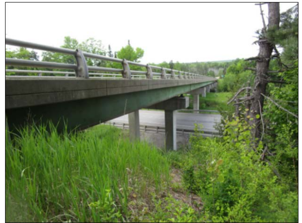
Casey Road/I-95 Interchange Bridge over Interstate 95 in Benedicta
