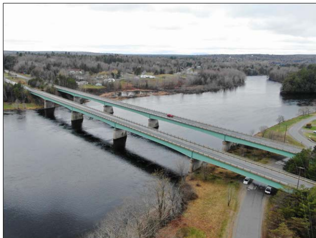
I-95 NB/SB over the Penobscot River - Vaughan Daggett Memorial Bridges
