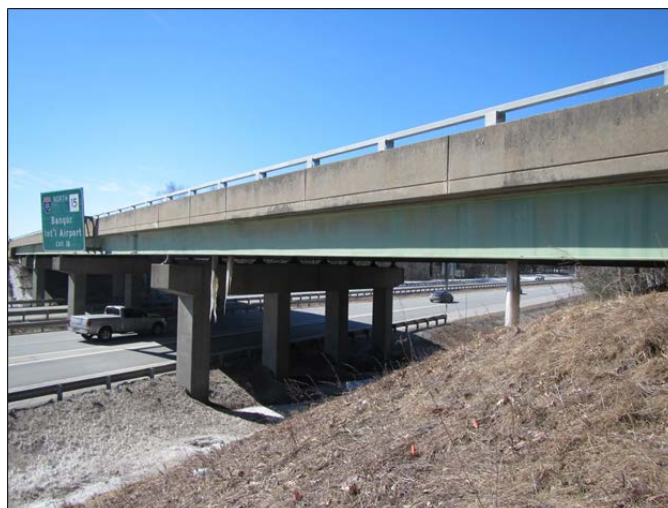
Route 202 over I-395 Bridge
