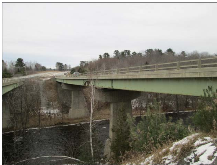
Route 202/Souadabscook Stream Bridges
