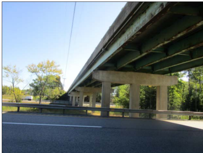
Route 155 /I-95 Interchange Bridge over Interstate 95 in Howland
