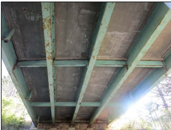
Photos 2 & 3: Route 155/I-95 Bridge – Scattered Cracking, Efflorescent Staining, and Delamination of Underside of Deck (left) and Deteriorated Substandard Bridge Rail (right)
