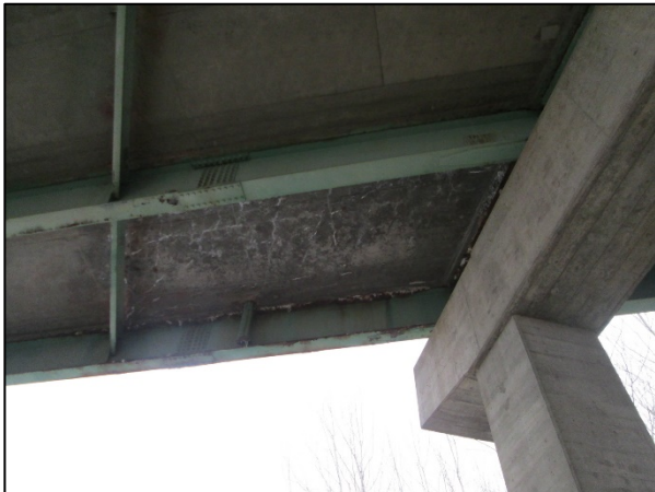
Photos 5 & 6: Route 202 over MCR Bridge – Deck Condition with Cracking and Efflorescence Staining (left) and Damaged and Leaking Deck Joint (right)
