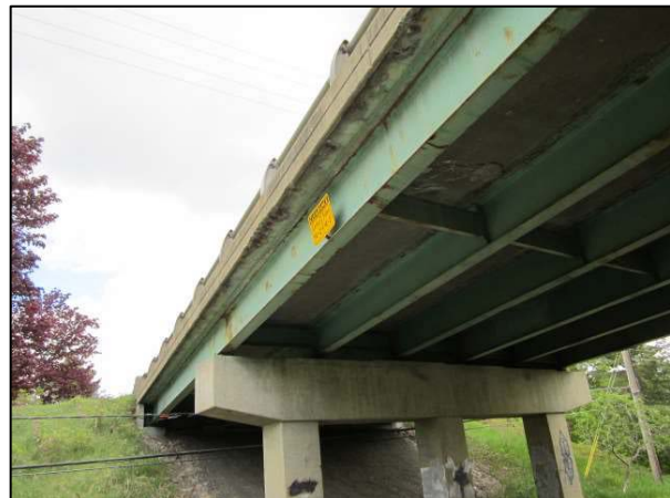
Photos 5 & 6: I-95 NB/SB over Route 116 Bridges – Deck Condition with Topside Cracking and Previous Patch Repair (left) and Deteriorated Deck Overhang (right)
