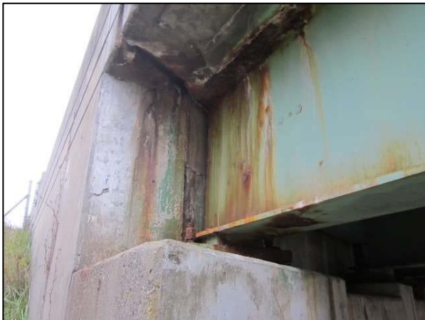
Photos 5 & 6: I-95 NB/SB over Webb Road Bridges – Poor Deck End and Backwall Condition due to Failed Deck Joint (left) and Deteriorated Deck Overhang (right)
