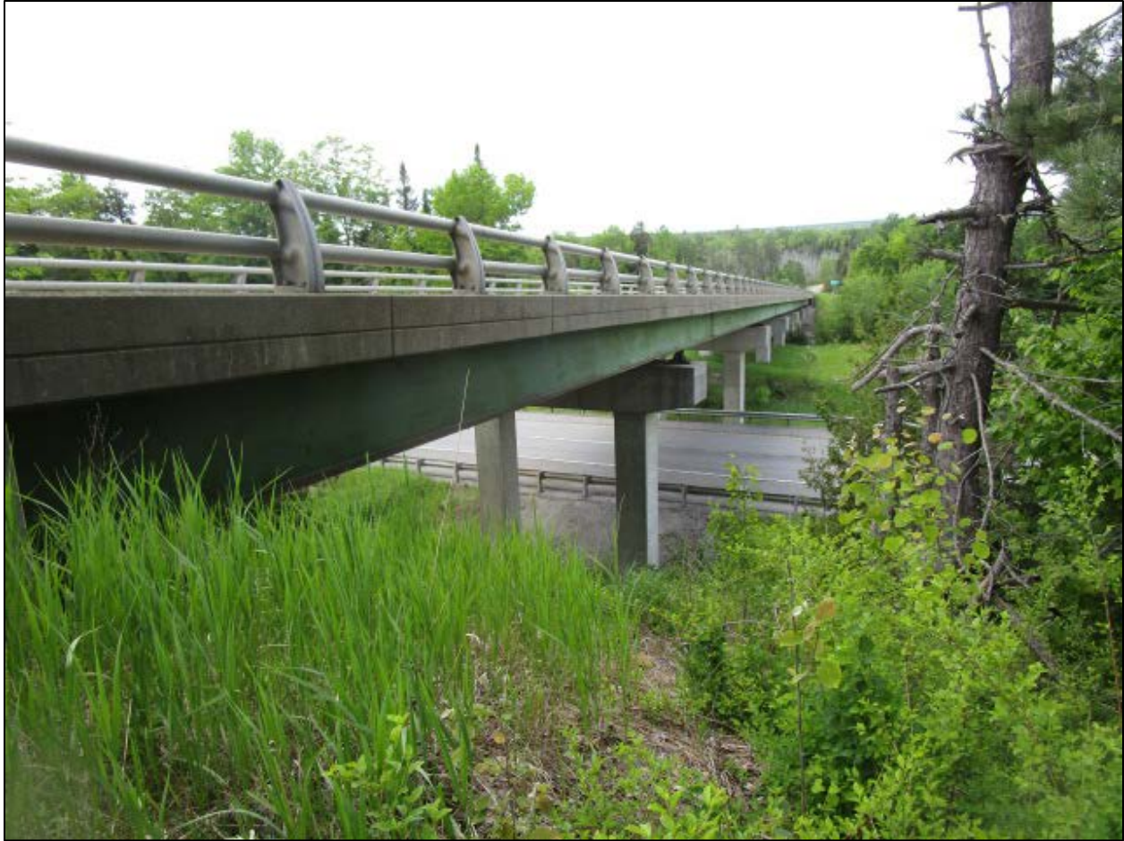
Photo 1: Casey Road/I-95 Interchange Bridge over Interstate 95
