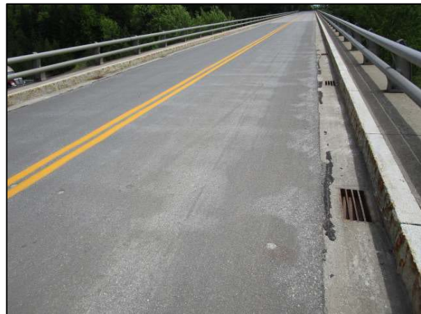
Photos 2 & 3: Casey Road/I-95 Bridge – Heavy Cracking and Efflorescent Staining of Underside of Deck (left) and Rutted Wearing Surface, Heavily Rusted Drains, and Substandard Bridge Rail (right)
