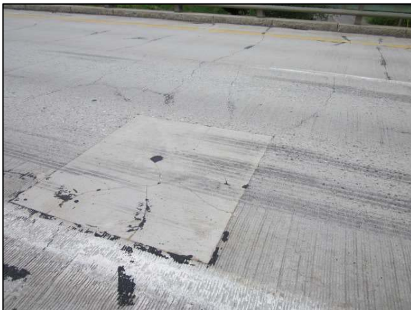
Photos 5 & 6: I-95 NB/SB over Route 116 Bridges – Deck Condition with Topside Cracking and Previous Patch Repair (left) and Deteriorated Deck Overhang (right)
