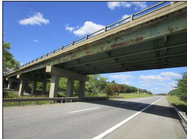
Photos 8 & 9: Route 157/I-95 Interchange Bridge – Deteriorated Condition of Deck Joint (left) and Deteriorated Deck Overhang (right)
