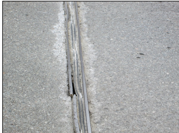
Photos 5 & 6: Route 202 over MCR Bridge – Deck Condition with Cracking and Efflorescence Staining (left) and Damaged and Leaking Deck Joint (right)
