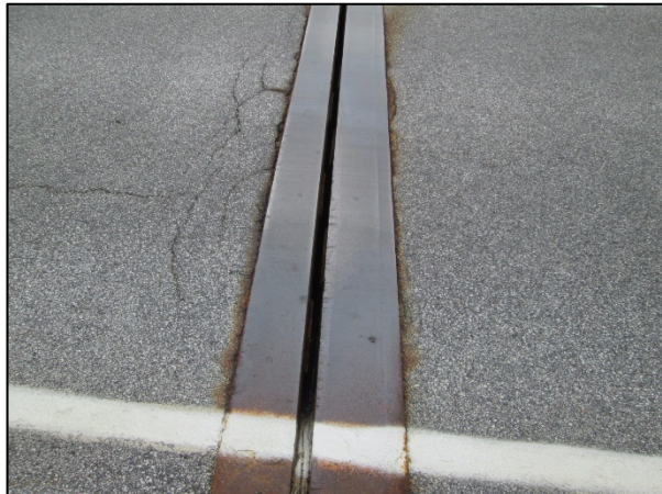
Photos 2 & 3: Route 202/Soudabscook Stream Bridges – Condition of Deck Underside with Cracking and Efflorescence Staining (left) and Failed Bridge Joint (right)
