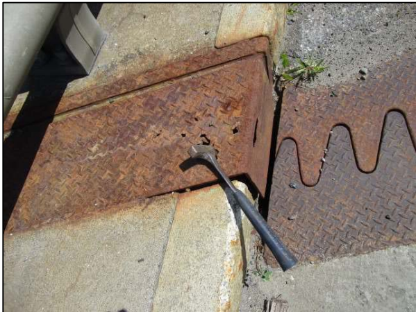
Photos 8 & 9: Route 157/I-95 Interchange Bridge – Deteriorated Condition of Deck Joint (left) and Deteriorated Deck Overhang (right)
