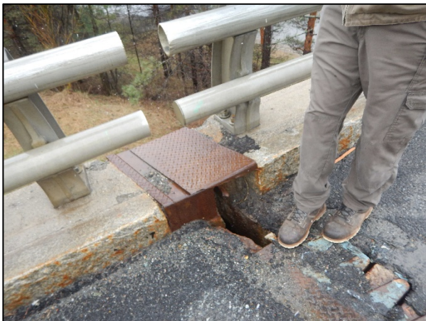
Photos 2 & 3: Vaughan Daggett Memorial Bridges – Condition of Deck Joint at North Abutment and Substandard Bridge Rail (left) and Deteriorated Deck Overhang (right)
