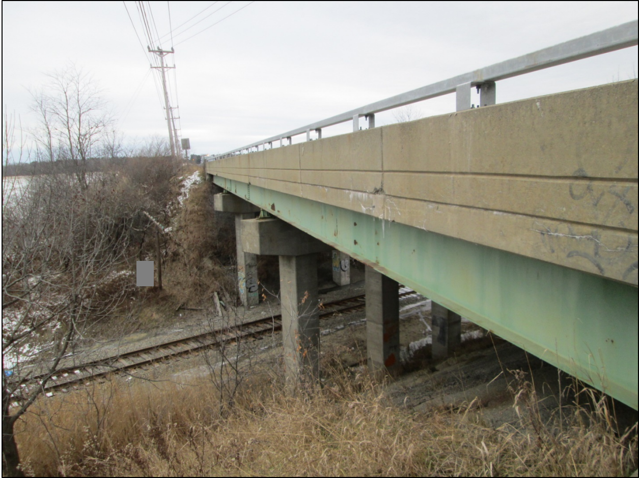
Photo 4: Route 202 over MCR Bridge
