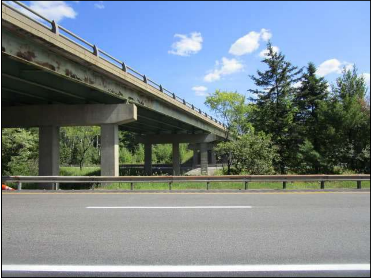
Photo 7: Route 157/I-95 Interchange Bridge
