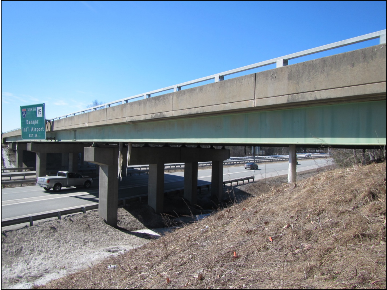
Photo 1: Route 202 over I-395 Bridge
