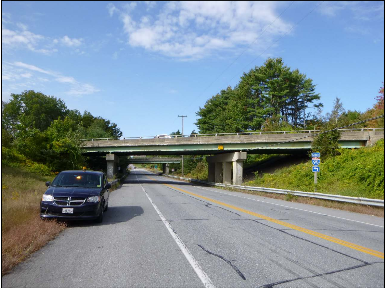
Photo 1: I-95 NB/SB over Somerset Avenue Bridges
