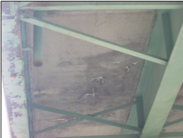
Photos 2 & 3: Route 202/Soudabscook Stream Bridges – Condition of Deck Underside with Cracking and Efflorescence Staining (left) and Failed Bridge Joint (right)
