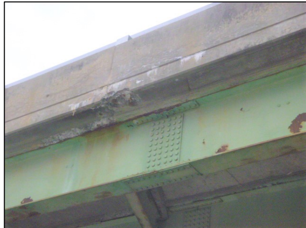
Photos 2 & 3: Route 202 over I-395 Bridge Numerous Deck Spalls over Travel Lanes of I-395 (left) and Spalled Deck Overhang (right)
