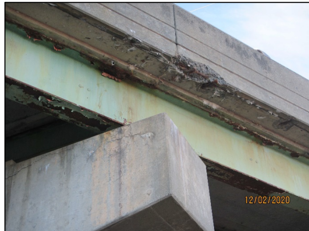
Photos 5 & 6: I-95 NB/SB over Webb Road Bridges – Poor Deck End and Backwall Condition due to Failed Deck Joint (left) and Deteriorated Deck Overhang (right)
