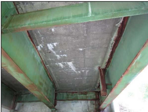
Photos 2 & 3: Casey Road/I-95 Bridge – Heavy Cracking and Efflorescent Staining of Underside of Deck (left) and Rutted Wearing Surface, Heavily Rusted Drains, and Substandard Bridge Rail (right)
