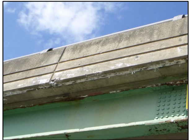
Photos 2 & 3: I-95 NB/SB over Somerset Avenue Bridges – Deteriorated Underside of Deck with Exposed Reinforcing Steel (left) and Deteriorated Deck Overhang with Delaminations and Excessive Efflorescent Staining (right)
