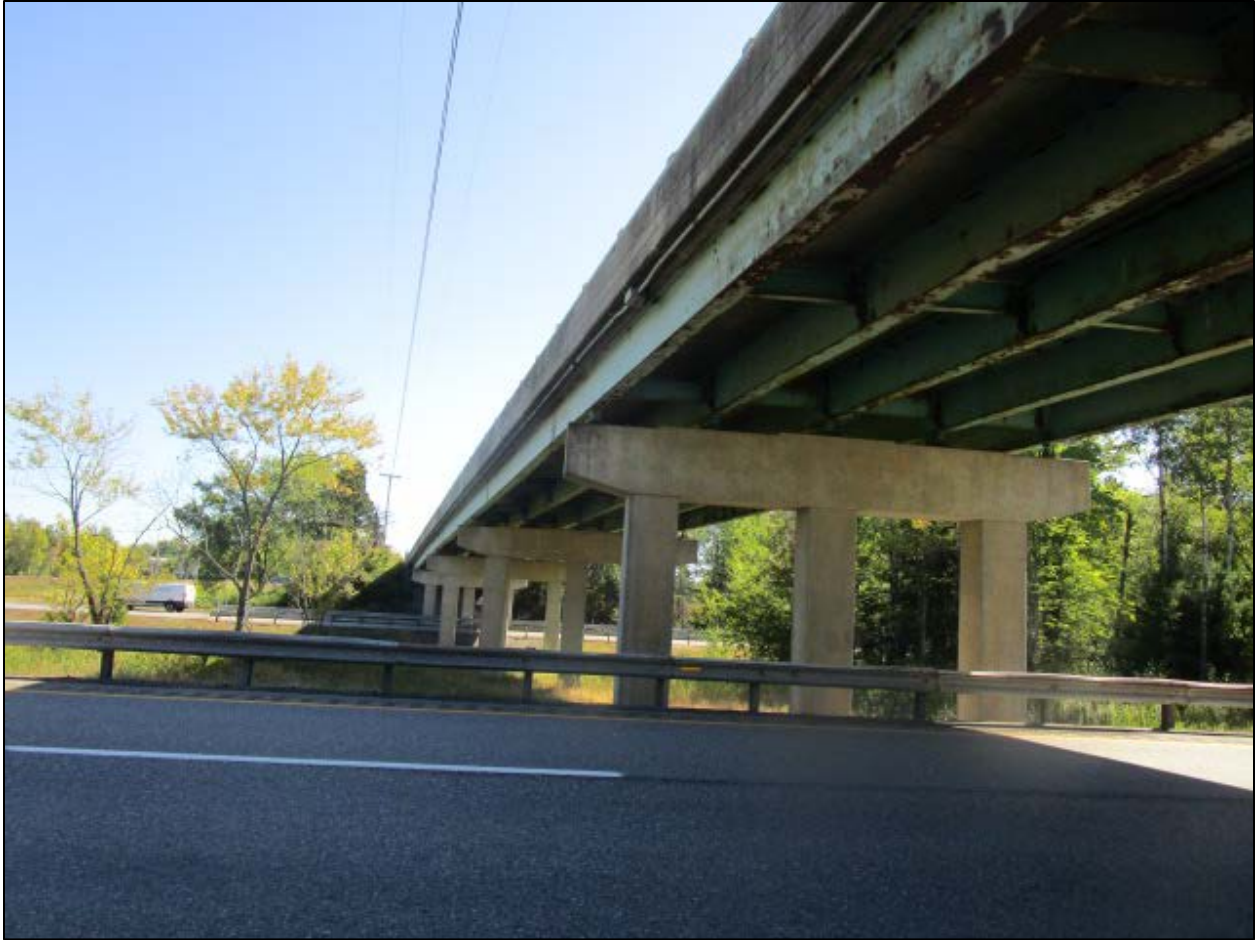
Photo 1: Route 155 /I-95 Interchange Bridge over Interstate 95
