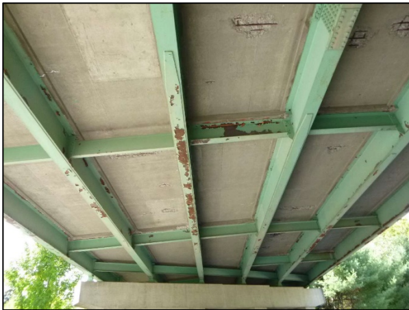
Photos 2 & 3: I-95 NB/SB over Somerset Avenue Bridges – Deteriorated Underside of Deck with Exposed Reinforcing Steel (left) and Deteriorated Deck Overhang with Delaminations and Excessive Efflorescent Staining (right)
