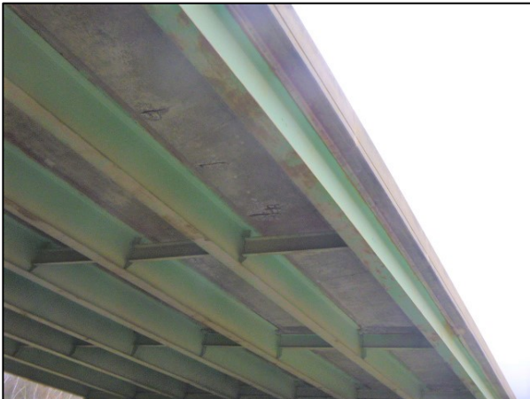
Photos 2 & 3: Route 202 over I-395 Bridge Numerous Deck Spalls over Travel Lanes of I-395 (left) and Spalled Deck Overhang (right)
