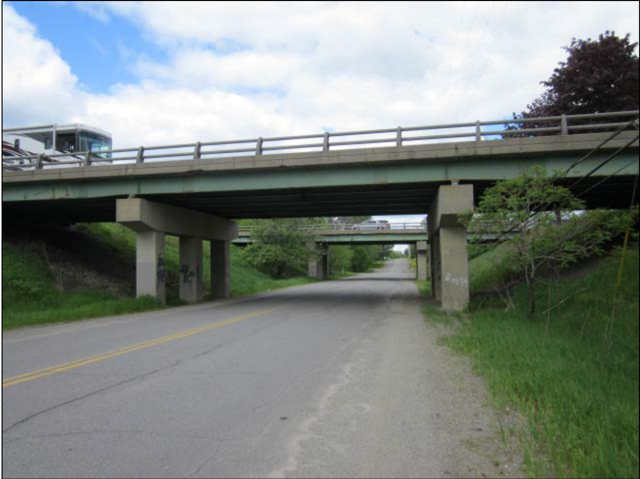
Photo 4: I-95 NB/SB over Route 116 Bridges
