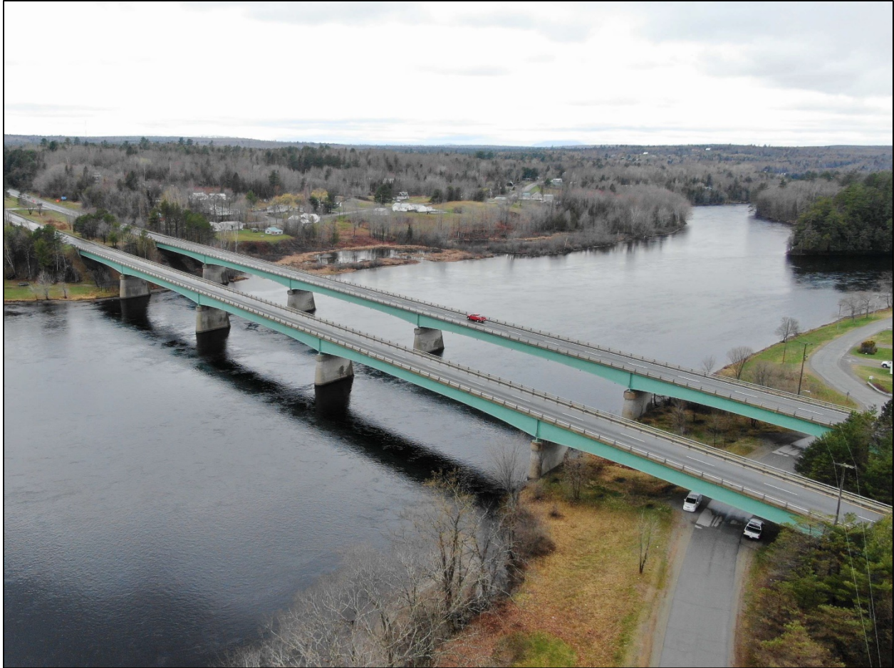
Photo 1: I-95 NB/SB over the Penobscot River - Vaughan Daggett Memorial Bridges
