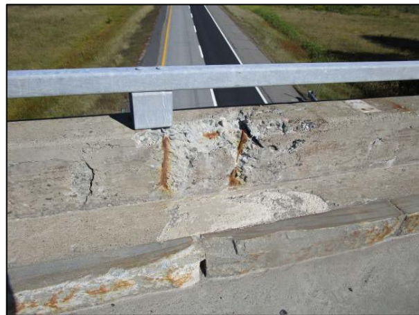
Photos 2 & 3: Route 155/I-95 Bridge – Scattered Cracking, Efflorescent Staining, and Delamination of Underside of Deck (left) and Deteriorated Substandard Bridge Rail (right)
