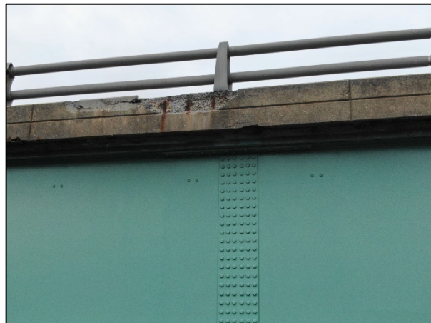
Photos 2 & 3: Vaughan Daggett Memorial Bridges – Condition of Deck Joint at North Abutment and Substandard Bridge Rail (left) and Deteriorated Deck Overhang (right)
