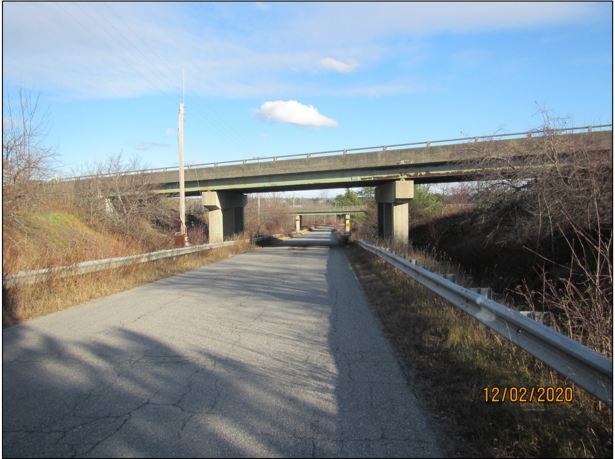
Photo 4: I-95 NB/SB over Webb Road Bridges
