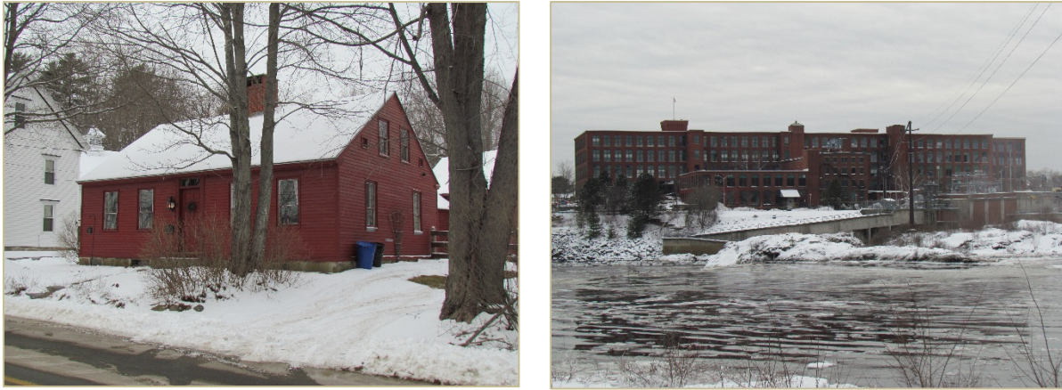
Figure 6. Left to Right: Summer Street Federal-era House and Cabot Mill
