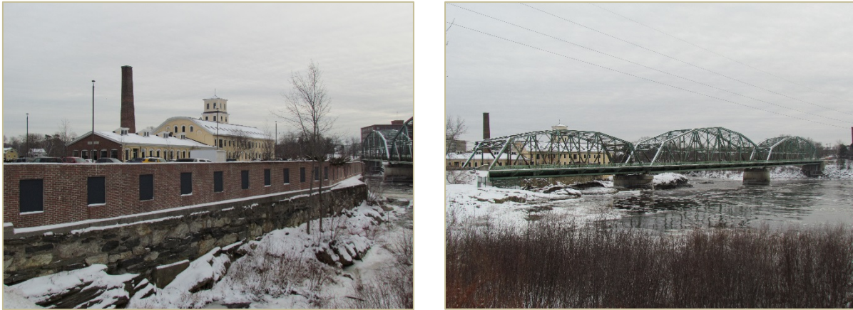
Figure 7. From Left to Right: Pejepscot Paper Company and Frank J. Wood Bridge
