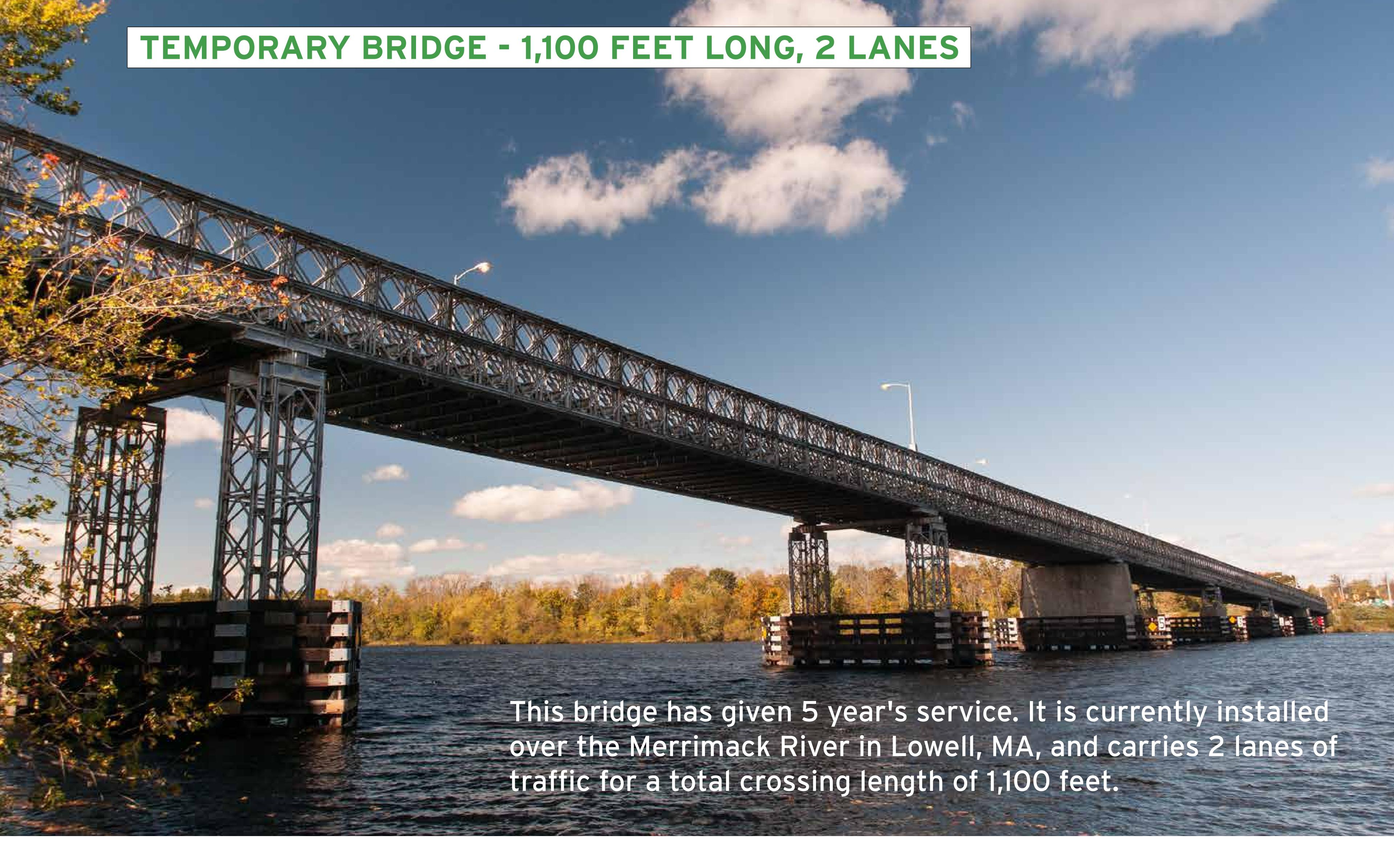
Misconception: The Road/Bridge will be closed for 2-3 years with Rehabilitation Truth: A temporary bridge is included in the 15M Rehabilitation Estimate. This is the fastest way to get full legal loads back on the crossing.
