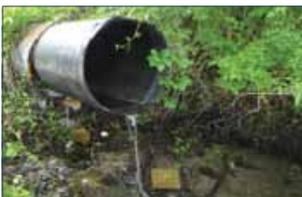
Inserting a smooth plastic liner inside an existing culvert may save money in the short term, but it raises water levels and increases flow velocities, which removes bed material and increases downstream scour. These problems make passage more difficult for fish and wildlife.
