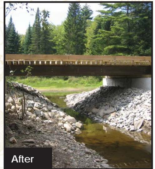
*The new bridge allows fish to pass at all flow levels.*
