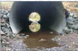
culvert properly embedded into streambed
