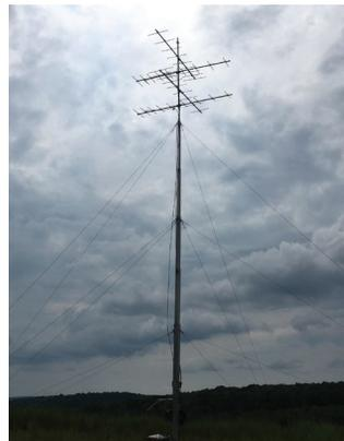
Figure 3b. A guyed, stand-alone tower array with two sets of quad-directional antennae.
