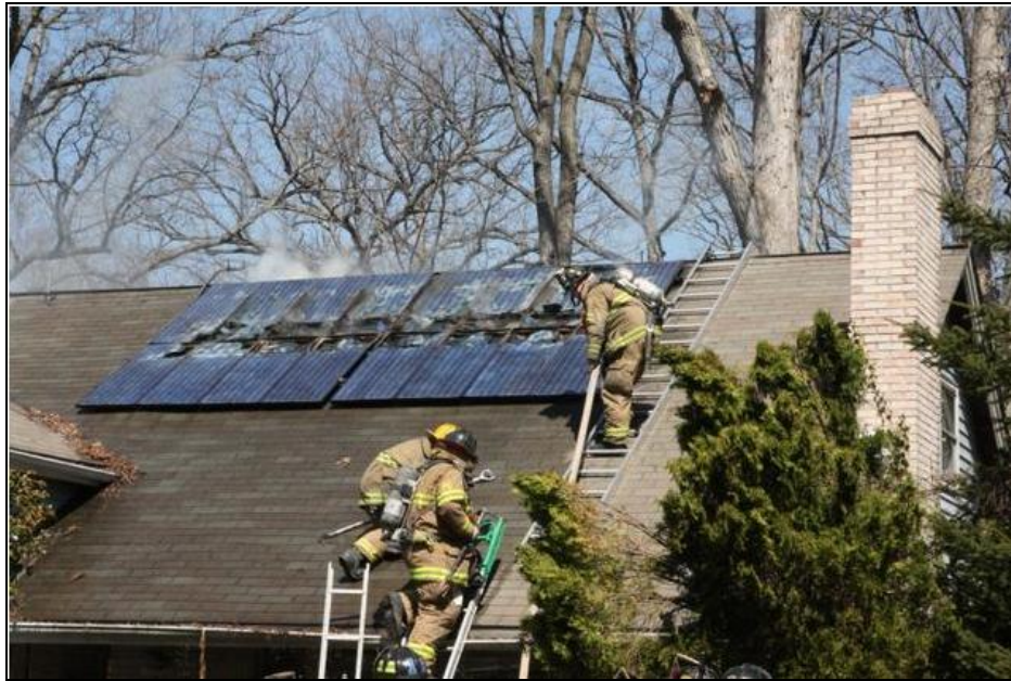
Figure 2-13: Residential PV Fire in March 2010 MD Incident 48
