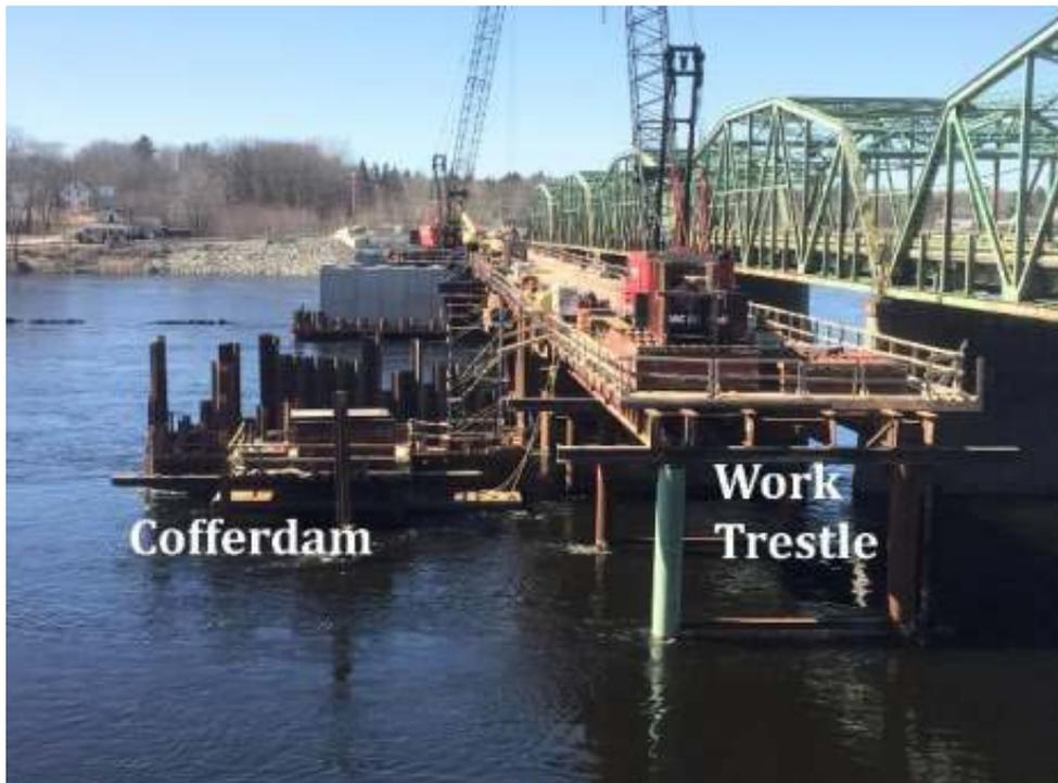
*Figure 2: Example of a pile-supported temporary work trestle adjacent to a sheet pile cofferdam*
