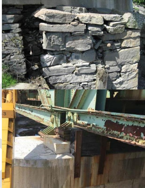
**Figure 16: Damaged concrete pedestals**
