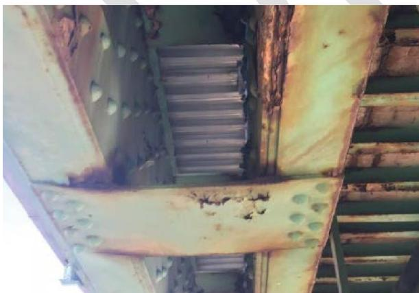
**Figure 12: Bottom chord lattice plate bowing**
