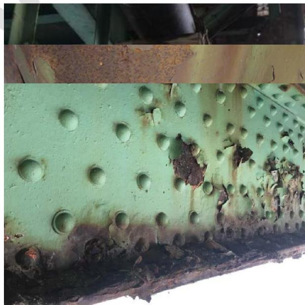
**Figure 11: Bottom chord bottom flange corrosion**
