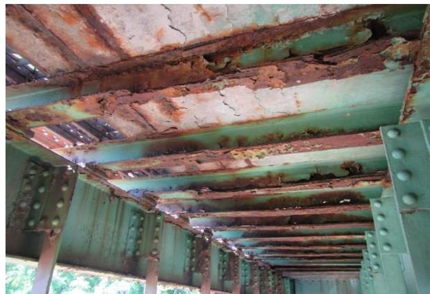
**Figure 8: Deteriorated crossbeams & deck**
