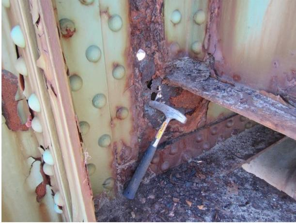
**Figure 9: Hole in floor beam**
