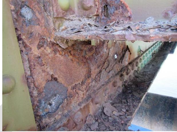
**Figure 10: Deteriorated floor beam**
