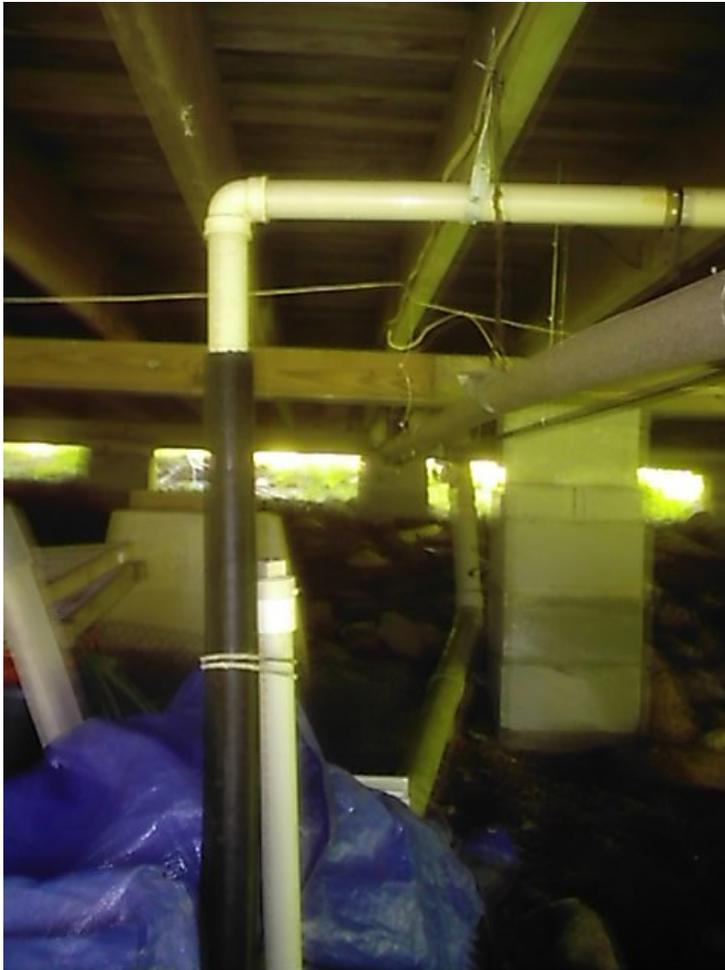
However, staff discovered that the drain line from the laundry room and kitchen sink had been cut, and the stub to the building drain had been capped. The greywater drain was connected to a black polyethylene pipe.
