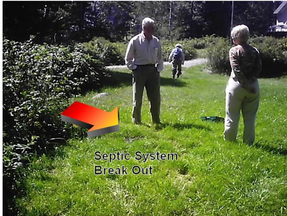
Adjacent to the nonconforming greywater disposal pit, there was evidence of an ongoing malfunction of the main disposal area. This was evident by a black, very wet area adjacent to an area overgrown with brush.
