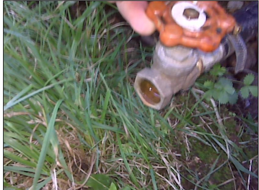
The main supply line from the well travels above grade and passes beneath the dwelling. This is the line below the utility room, showing the PEX tubing supply line going into the dwelling. The end of main line ends in a gate valve used to drain the line for the winter. Note the moisture in the end of the valve, and the valve's position on the ground.
