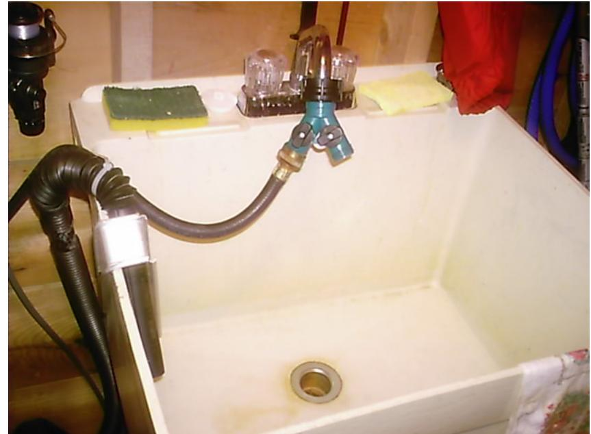
Plumbing fixtures inside the dwelling were examined for potential cross connections. The photograph on the left shows where the potable water supply enters the building through the floor of the utility room. The photograph on the right shows the water supply and discharge of a laundry machine in the utility room.
