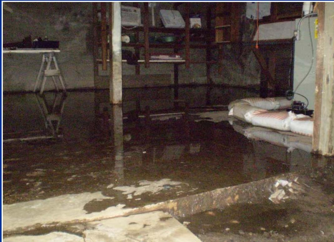
Seepage of effluent into parts of buildings below ground or back-up of wastewater into the building.
