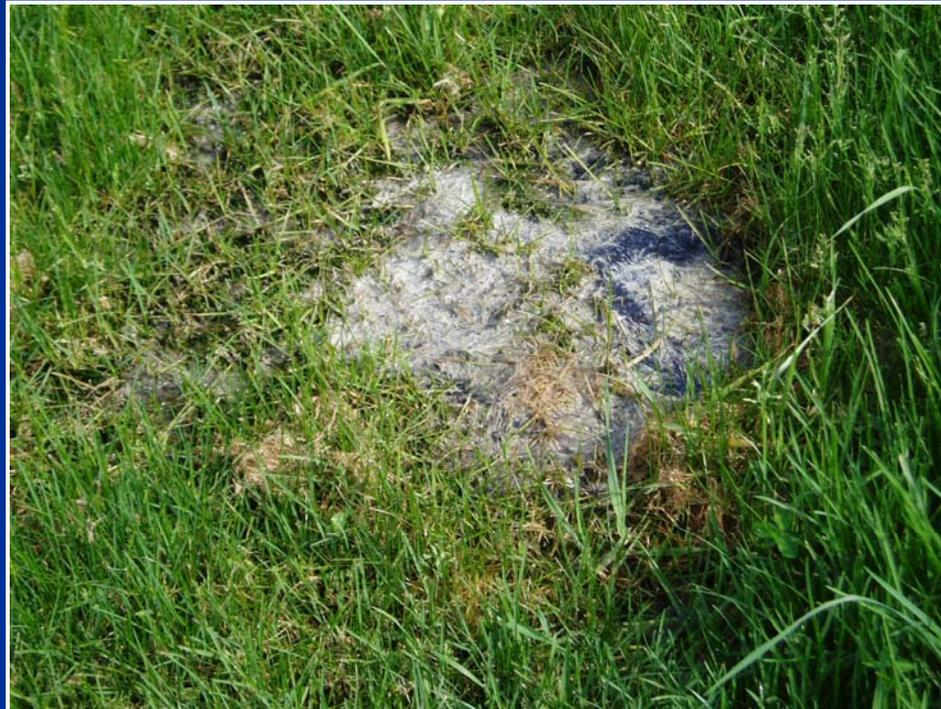
Ponding or outbreak of wastewater or septic tank effluent onto the surface of the ground.
