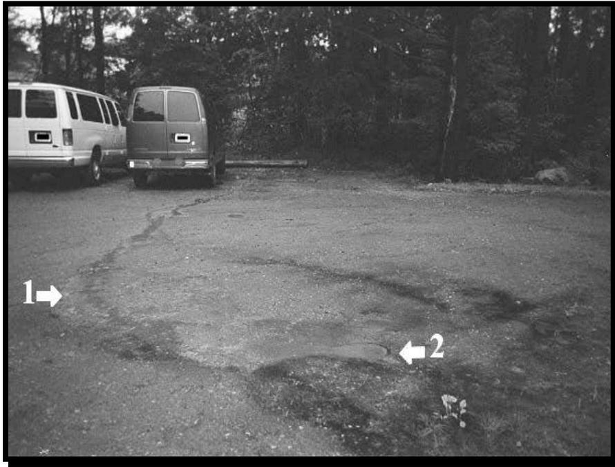
**Figure 68. Malfunction resulting in effluent runoff (1) and breakout (2).**
