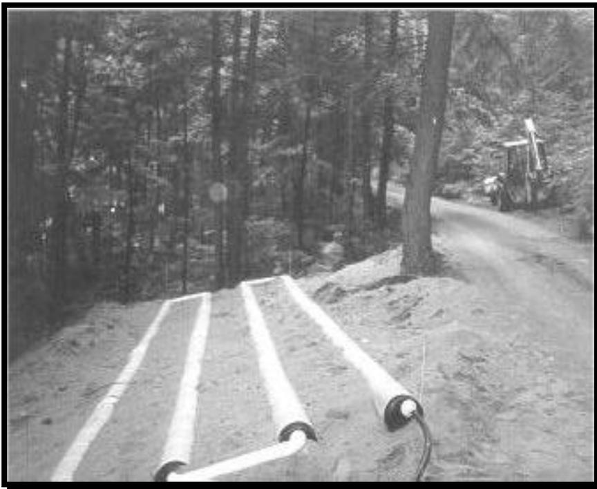
**Figure 16. Fabric covered tubes installed for serial distribution.**
