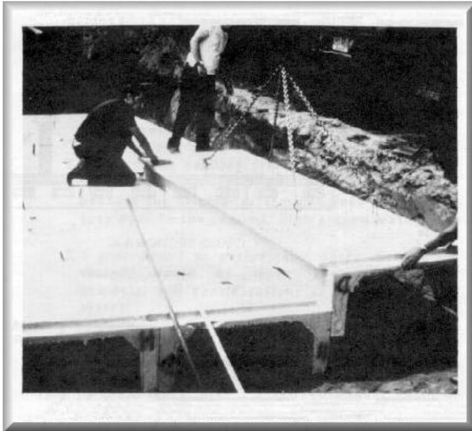
**Figure 8. Concrete chamber system during construction**
