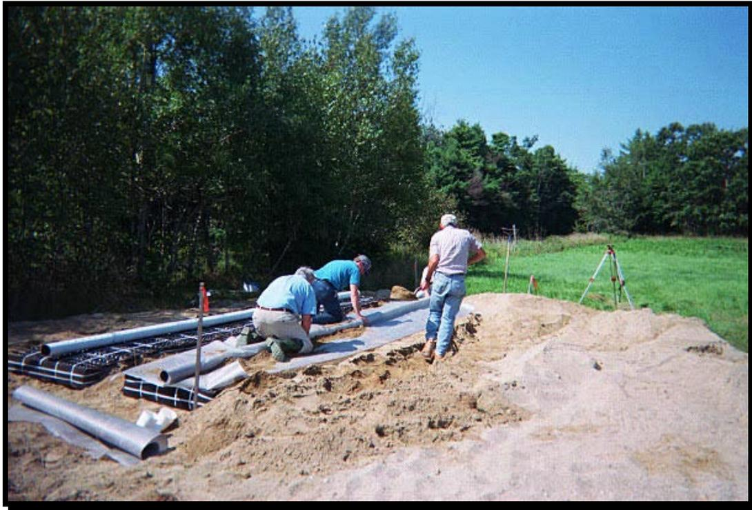
**Figure 18. Installation of a cusped block gravel-less bed.**
