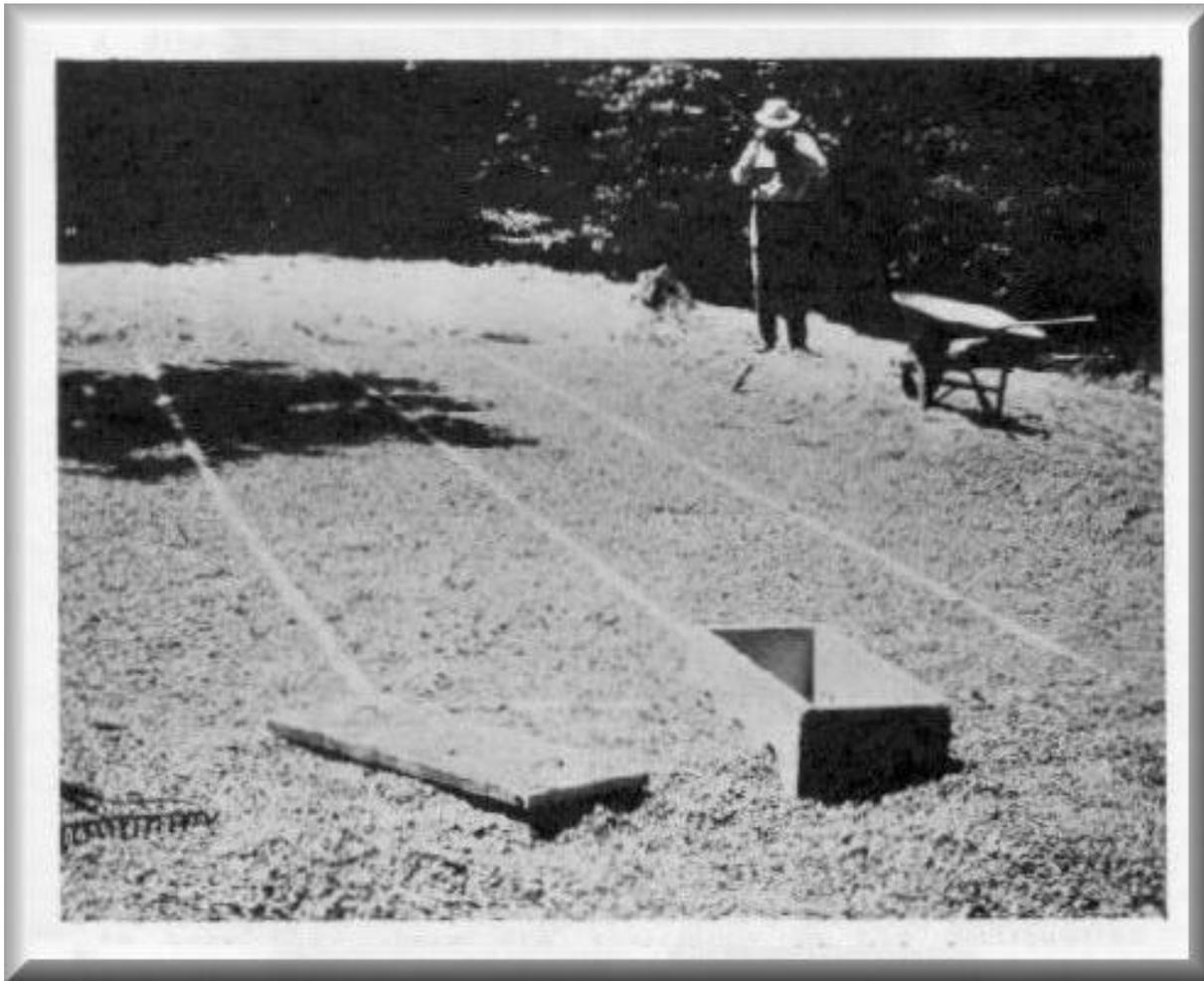
**Figure 5. Stone layer of disposal bed during construction**
