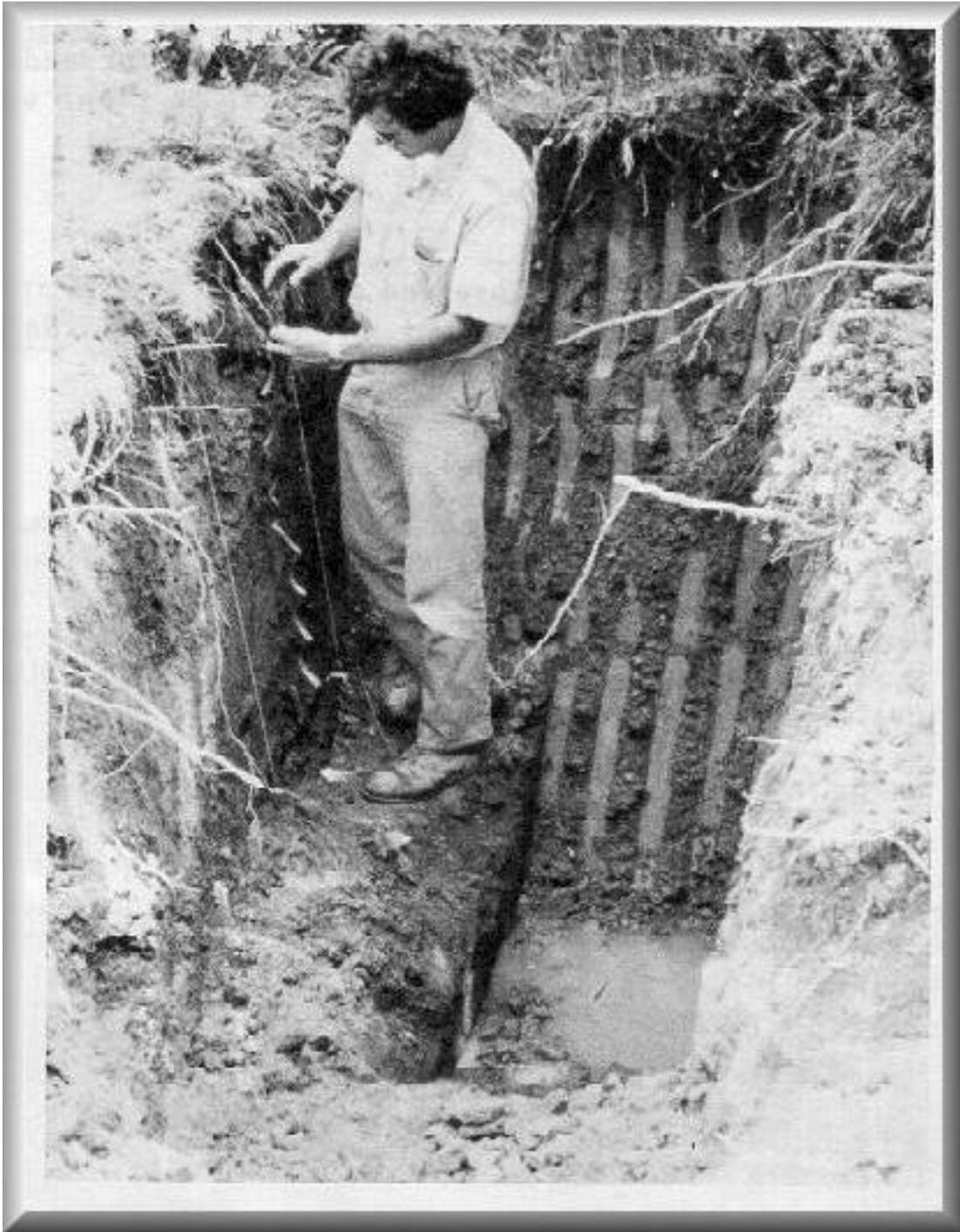
**Figure 37. Test pit excavated with a backhoe to a depth of four feet**
