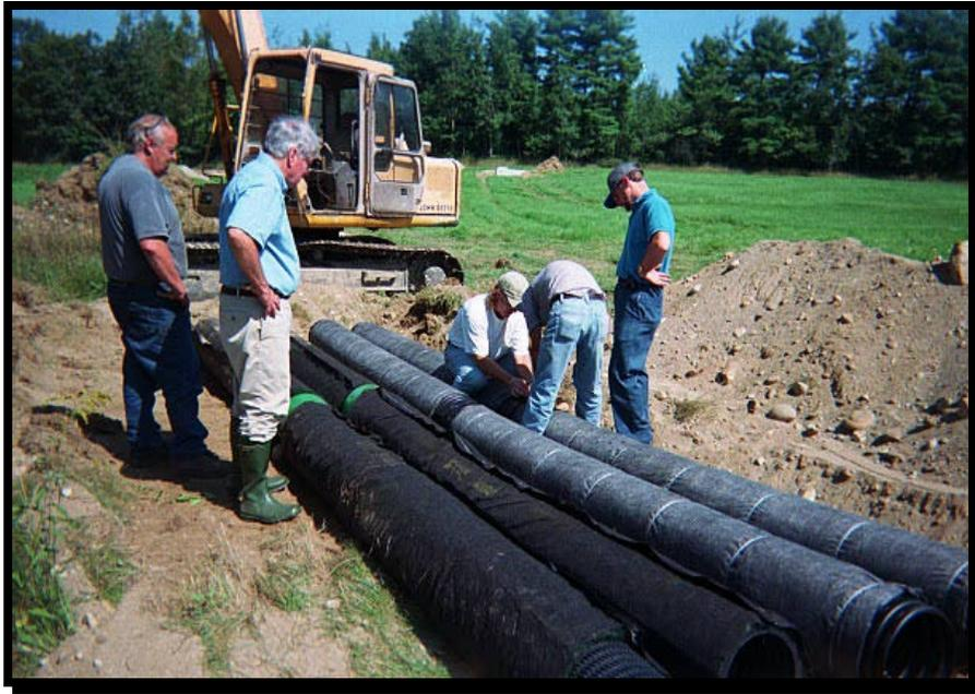
**Figure 15. Fabric covered tube installation.**
