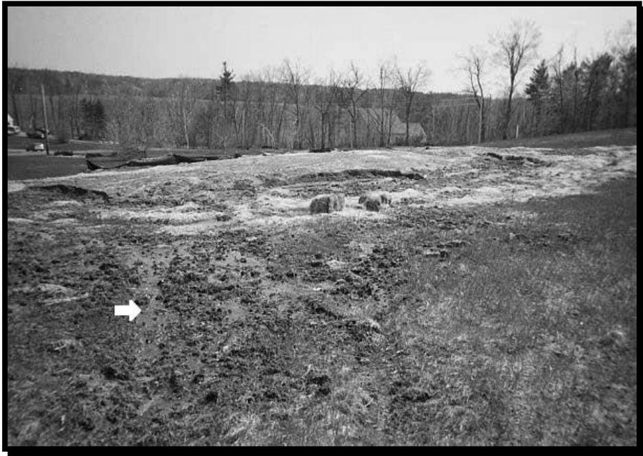
**Figure 67. Malfunction resulting in effluent breakout and ponding (arrow).**
