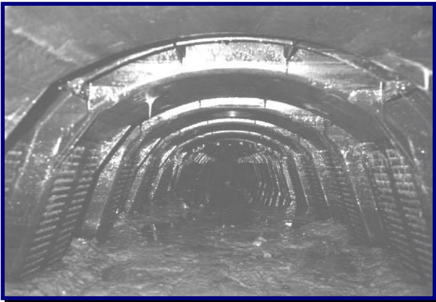
**Figure 12. Plastic chamber installation showing interior and established biomat.**
