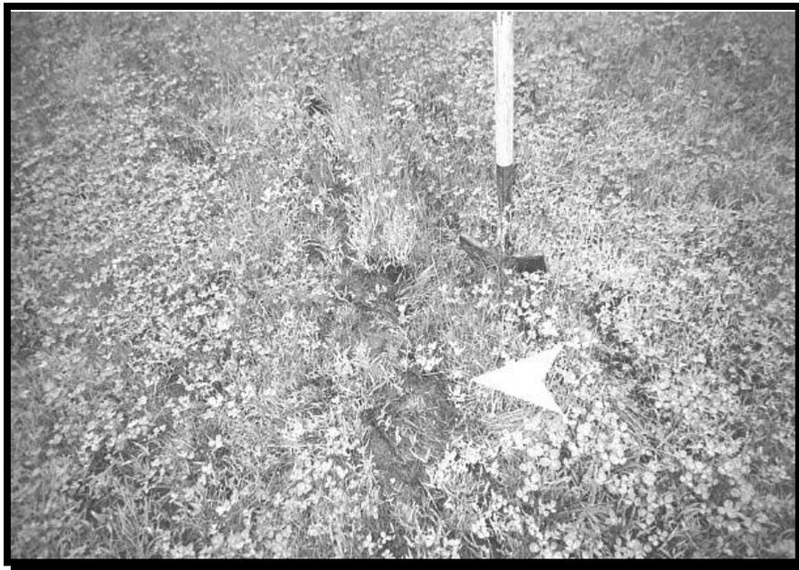
**Figure 69. Malfunction resulting in a chronic wet area (arrow).**
