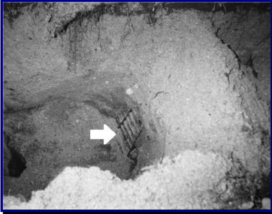
**Figure 11. Plastic chamber installation showing exposed sidewall and back fill.**
