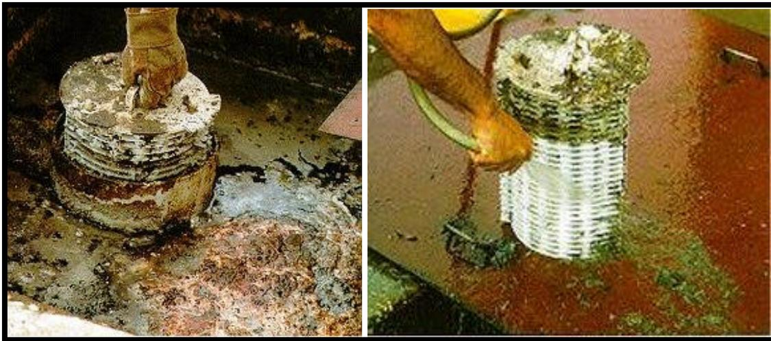
**Figure 26. Solids being removed from an outlet filter.**
