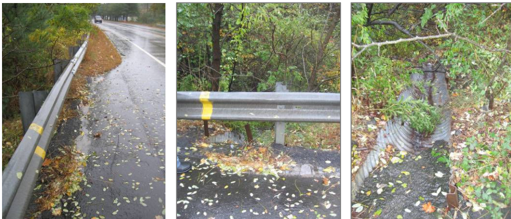
Site 3 Photos: Stormwater from Industrial Parkway drains to a road curb cut (left and middle) which leads to a metal half-culvert (right) that channels water to the stream.
