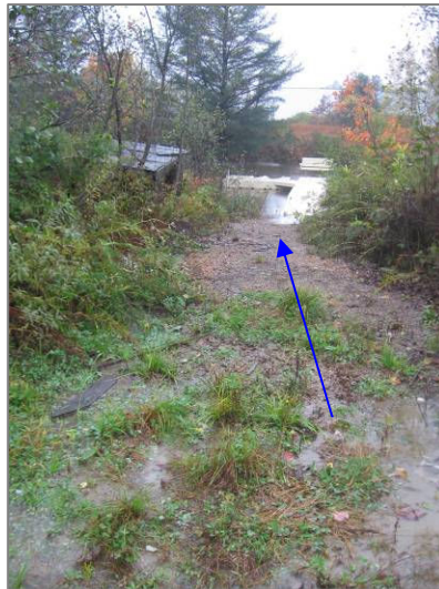
Site 2A Photos: A storm drain surrounded by unstabilized soil drains the unpaved lot, delivering sediment and debris to the stream (left). Portions of the unpaved lot drains through an unvegetated passage directly to the stream (right).
