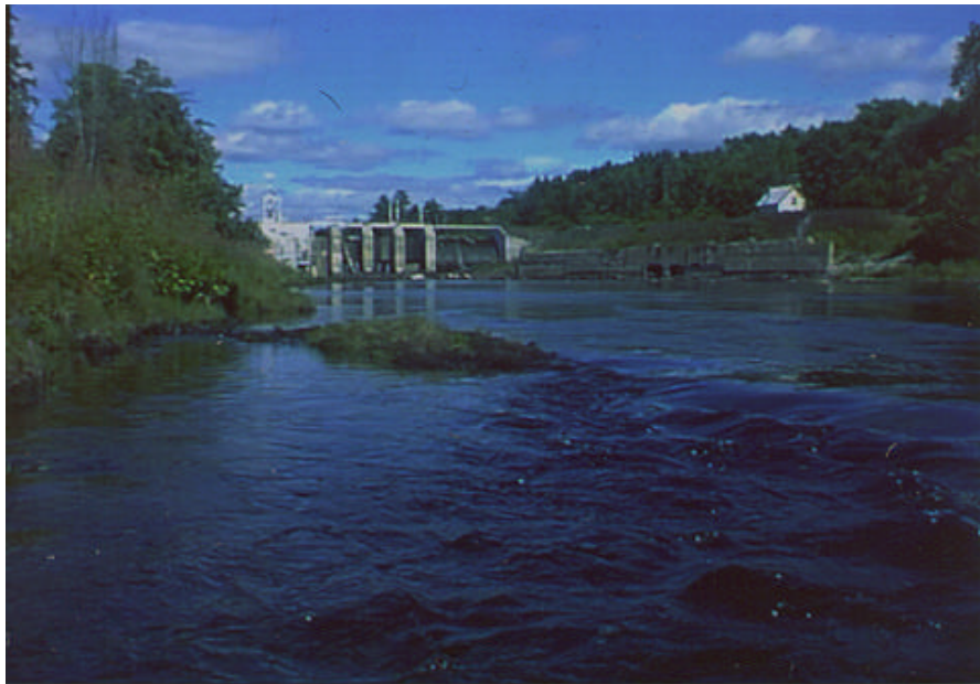
Benton Falls Dam, Sebasticook River, Benton , Maine
