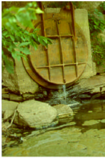
Combined Sewer Overflow discharging to the Androscoggin River in Auburn (1984, approx.)
