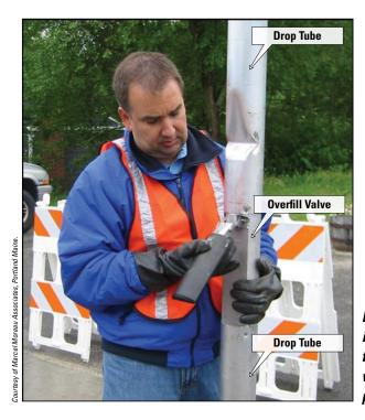
tube that releases a valve, or flapper, inside the tube when the liquid level in the tank reaches 95% of full-tank volume. When this happens, the product flowing down the fill pipe slams the valve shut, severely restricting flow of fuel into the tank. The delivery hose "jumps," alerting the driver that the flapper has closed. At this point, the driver should stop the flow of fuel from the truck and drain any
