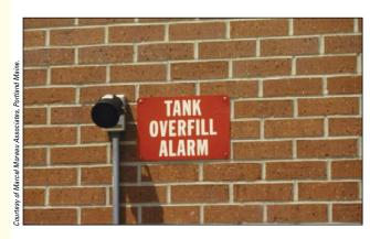
Here is a different type of overfill alarm that is labeled so the delivery driver knows that when it sounds, it is talking to him.
