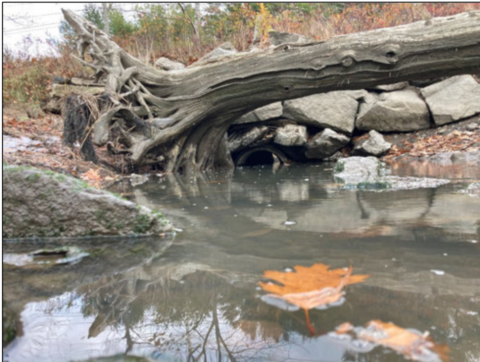
Photo 4: Culvert Outlet with Dry-Laid Stone Headwall (Photo Taken 11/11/2020)
