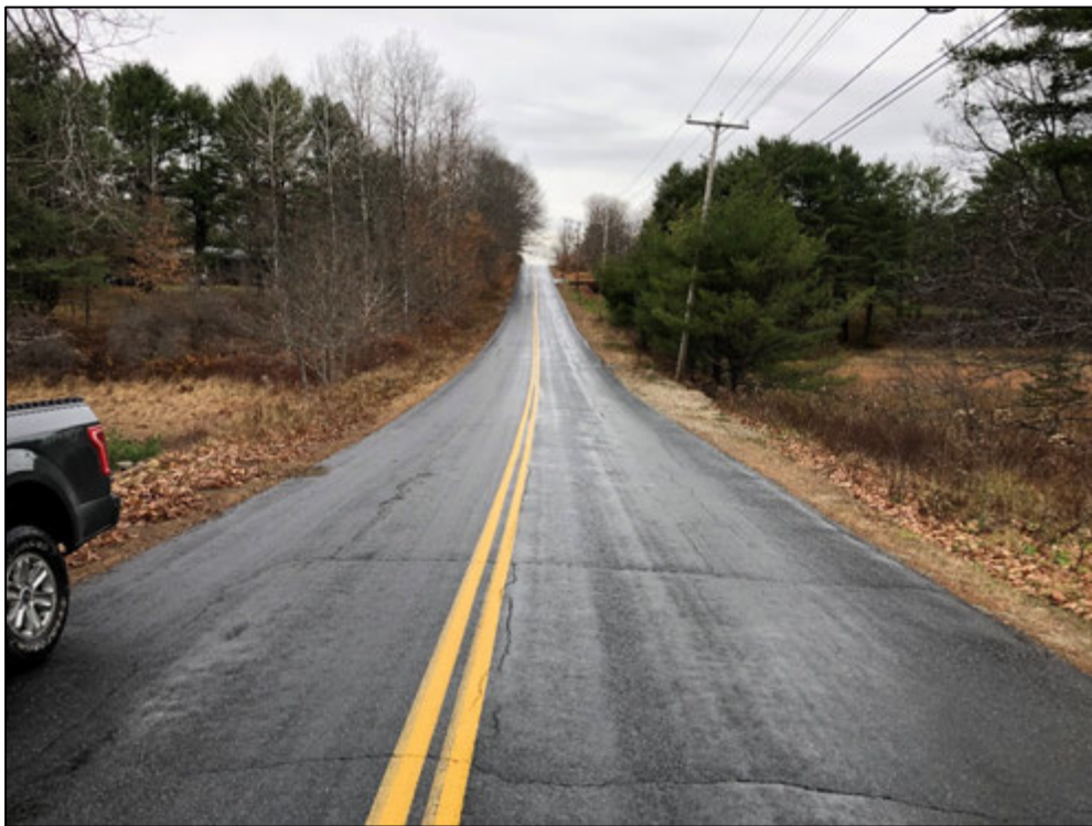
Photo 10: Old Ferry Road at Crossing (Photo Taken 11/12/2020)
