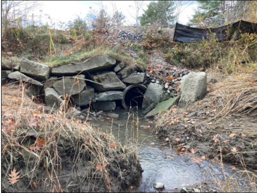
Photo 3: Culvert Inlet with Dry-Laid Headwall (Photo Taken 11/11/2020)
