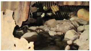
Figure 4 Void between the culverts
