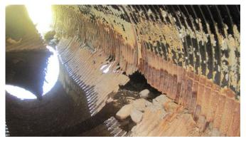
Figure 2 Showing holes allowing rocks to enter culvert
