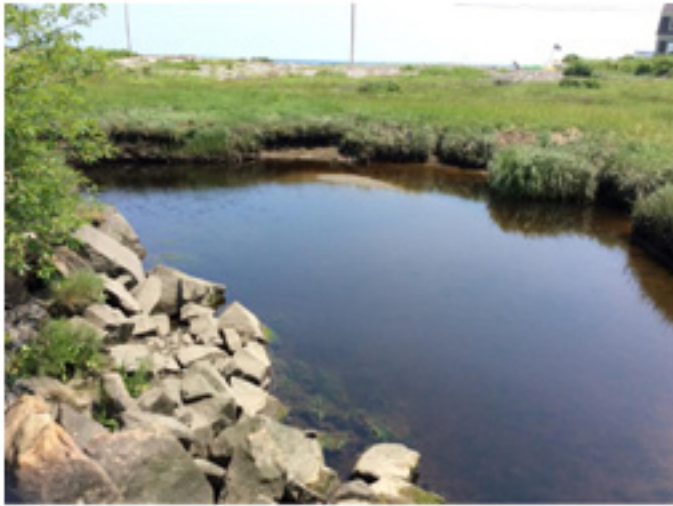
VIEW: Upstream of Inlet DATE TAKEN: July 10, 2015
