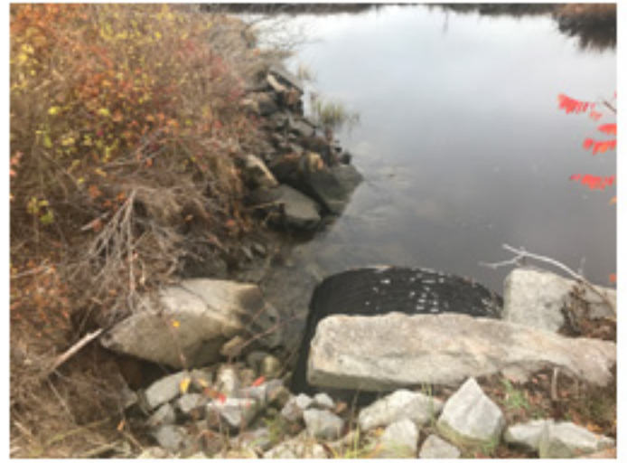
VIEW: Inlet End of Culvert DATE TAKEN: October 29, 2019
