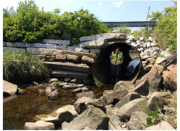
VIEW: Inlet End of Culvert DATE TAKEN: July 10, 2015
