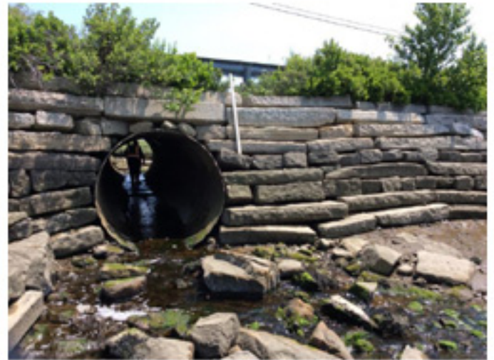
VIEW: Outlet End of Culvert DATE TAKEN: July 10, 2015
