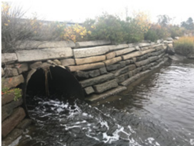
VIEW: Outlet End of Culvert DATE TAKEN: October 29, 2019
