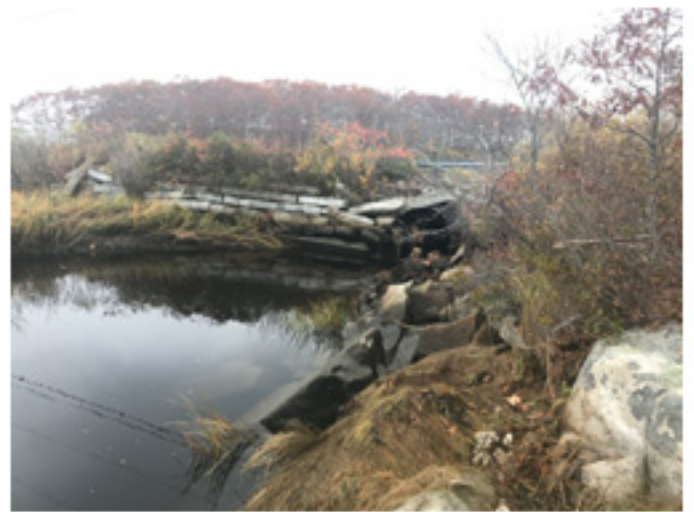
VIEW: Inlet End of Crossing DATE TAKEN: October 29, 2019
