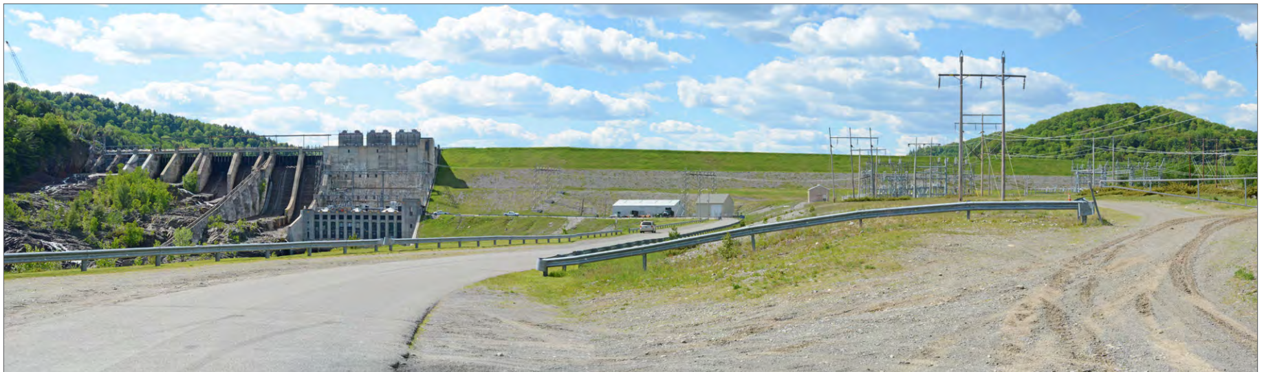
P31. Panoramic view looking east to northwest toward the Wyman Hydroelectric Dam. The closest proposed turbine is 4.4 miles away and will not be visible from this location due to intervening terrain and foreground vegetation.
