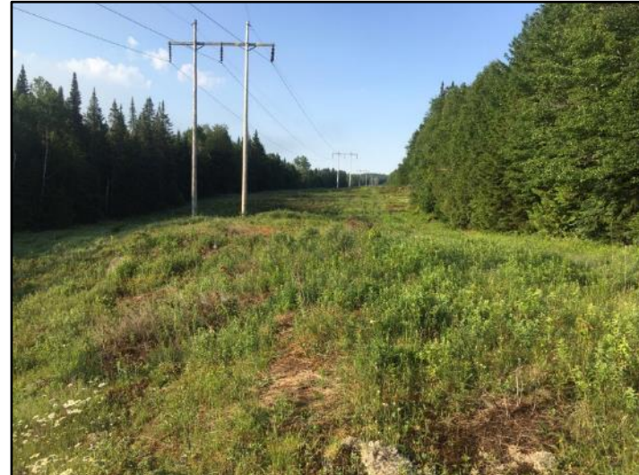
10: UPSA-4 West, T-line at bend, 7/2/20
