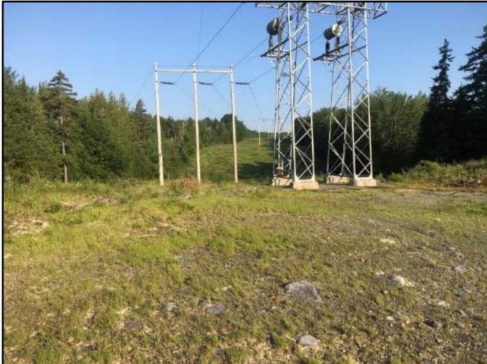
9: UPSA-4 North, T-line at bend, 7/2/20
