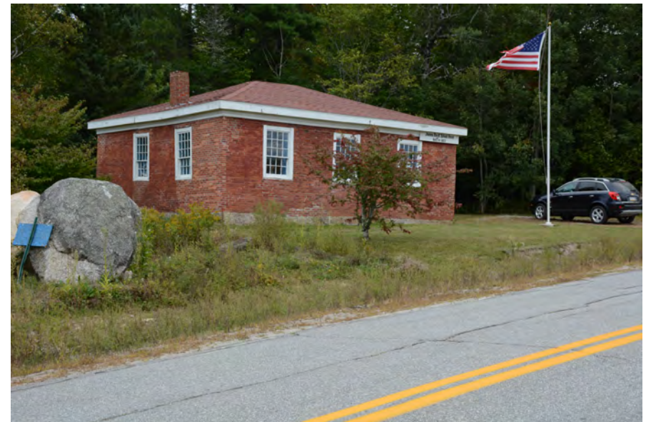
View looking southeast at the Brick School House, built in 1827. The structure now houses a museum open on Sundays. The Project will not be visible from the schoolhouse due to intervening vegetation behind the structure.
