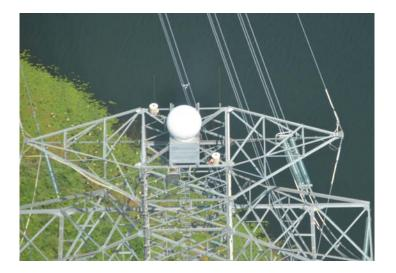
Figure 4. DeTect X-Band ADLS Radar With Radome Enclosure
