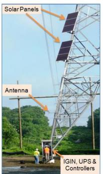
Figure 2: Typical ADLS Site on Susquehanna-Roseland Line on fiber/radio hybrid network.
