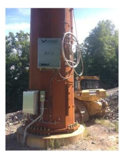
Figure 15. The DCU Installed on Transmission Tower [6]
