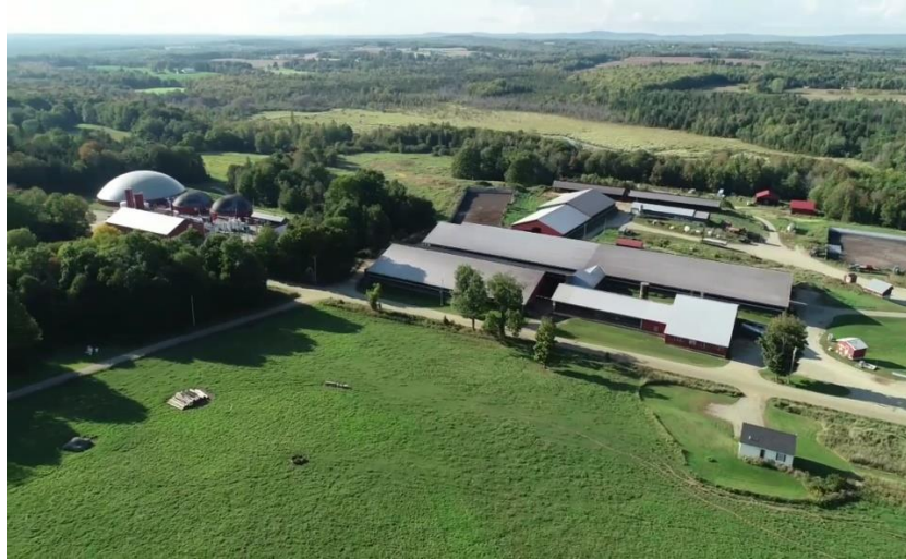
Exeter Agri-Energy - Plant Overview
