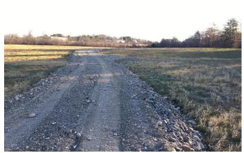
Photo 20 (11/12/18): View, looking east, of the gravel road constructed in the Site hayfield for drill rig access.
