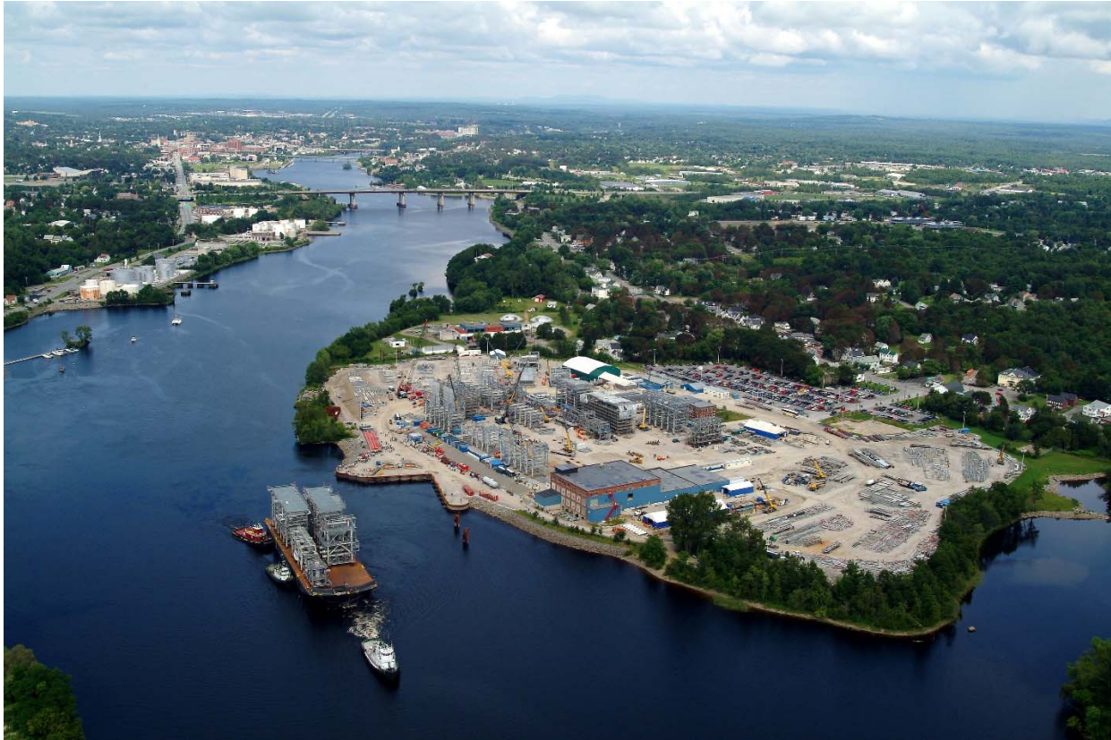
Figure 1 – Offsite Staging Area; Cianbro's Eastern Manufacturing Facility in Brewer, ME
