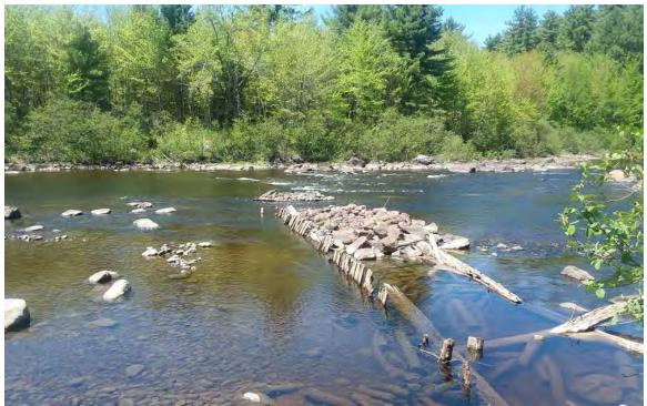
PHOTO 5-6 RELIC CRIBWORK LIKELY FROM HISTORIC LOGGING OPERATIONS SPANS THE WIDTH OF THE DEAD RIVER UPSTREAM FROM GRAND FALLS
