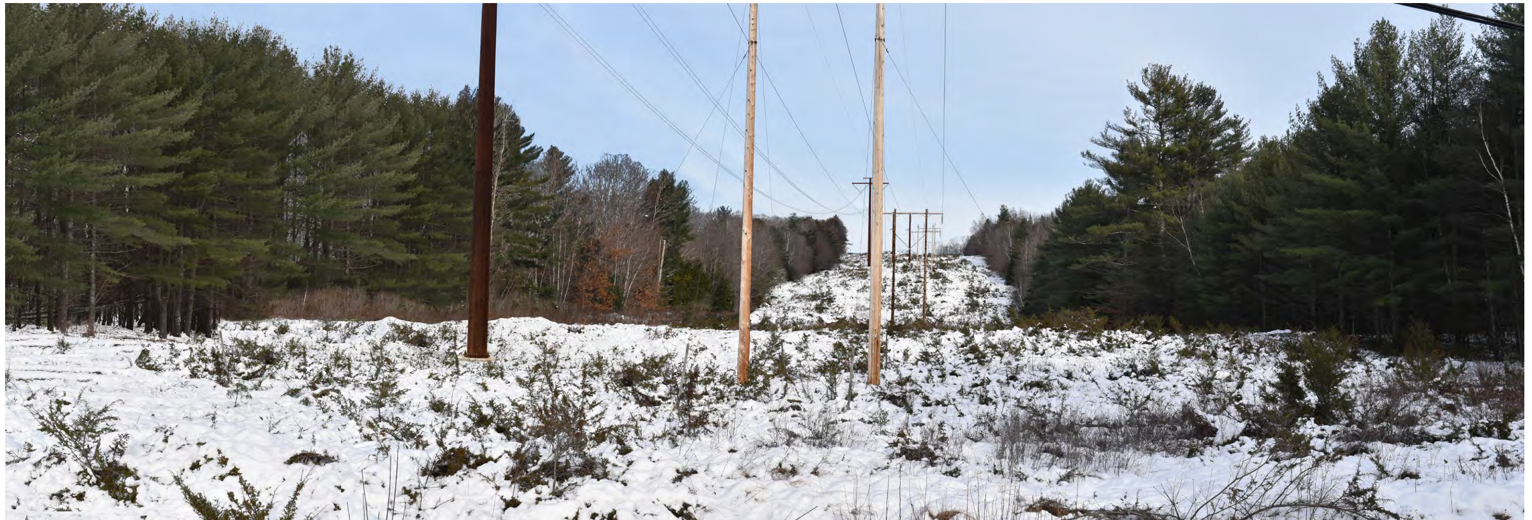
Proposed Conditions: Panoramic view looking from north to east from Route 201 in Moscow toward the proposed co-located HVDC transmission line. The existing 225 ft wide corridor clearing will be widened by 75 ft on the western side (left of corridor in image) to accommodate the proposed transmission line. Three structures will be visible from this viewpoint.
