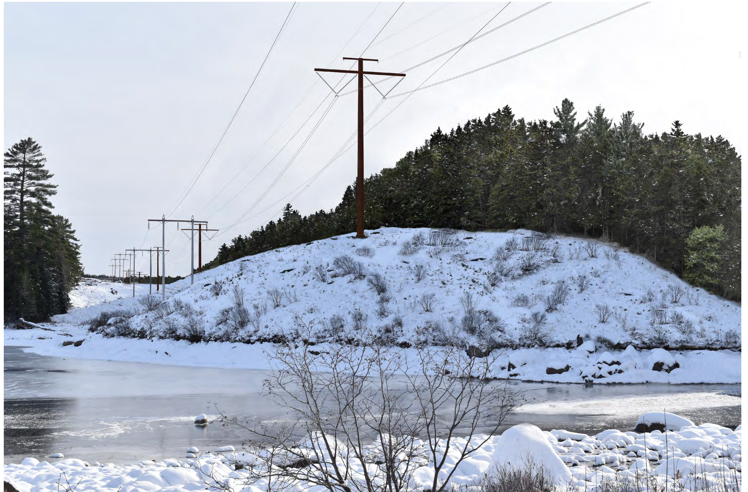
Proposed Conditions: Normal view looking south on Troutdale Road (private road) looking toward the proposed co-located HVDC transmission line. The existing 150 ft wide transmission line clearing will be widened by 75 ft on the western side to accommodate the new HVDC transmission line corridor. Portions of six proposed HVDC structures will be visible from this viewpoint.
