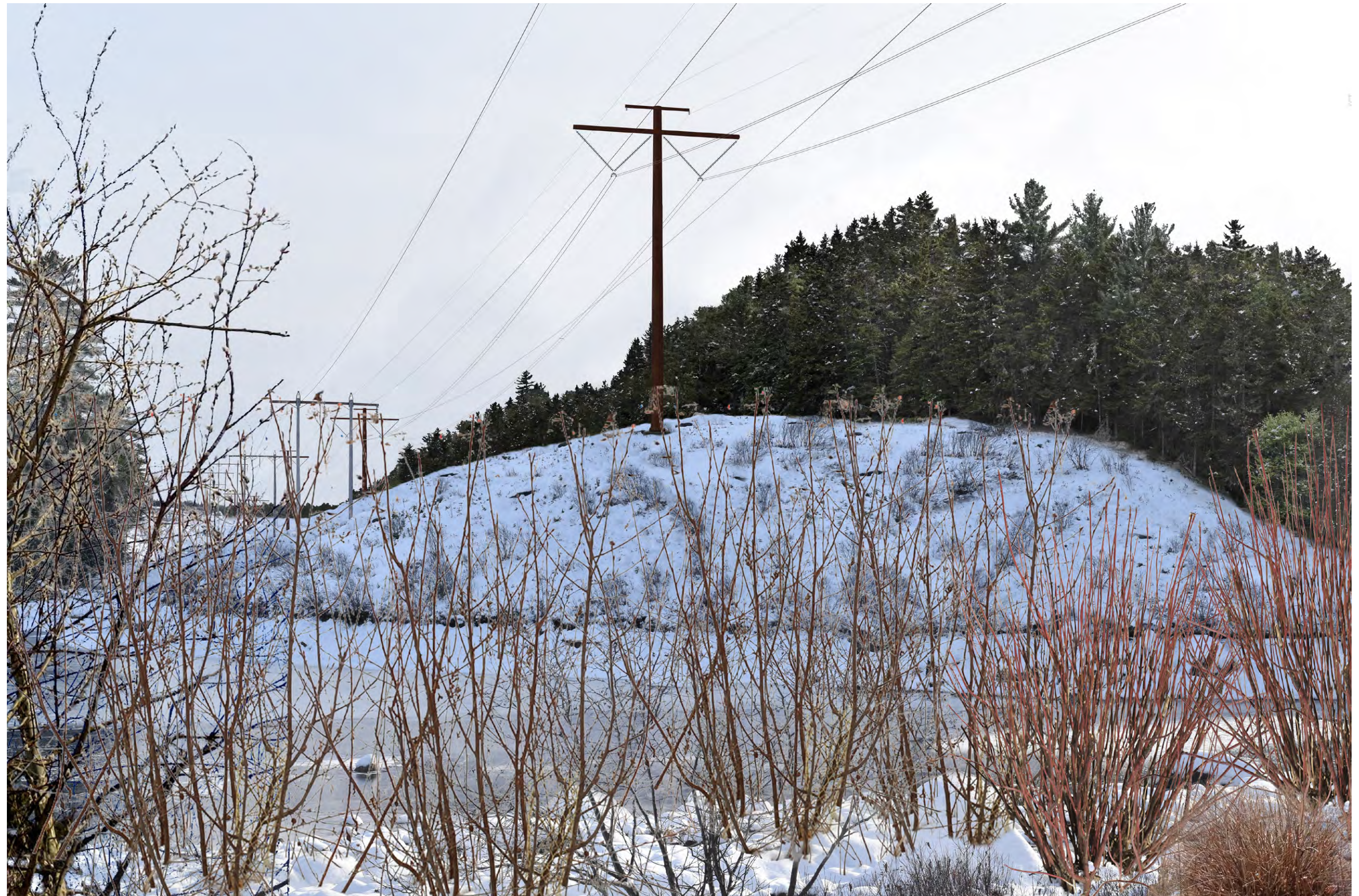
Proposed Conditions: Normal view looking south on Troutdale Road (private road) looking toward the proposed co-located HVDC transmission line with proposed Joes Hole (Moxie Pond) buffer plantings in the foreground . The existing 150 ft wide transmission line clearing will be widened by 75 ft on the western side to accommodate the new HVDC transmission line corridor. Portions of six proposed HVDC structures will be visible from this viewpoint.
