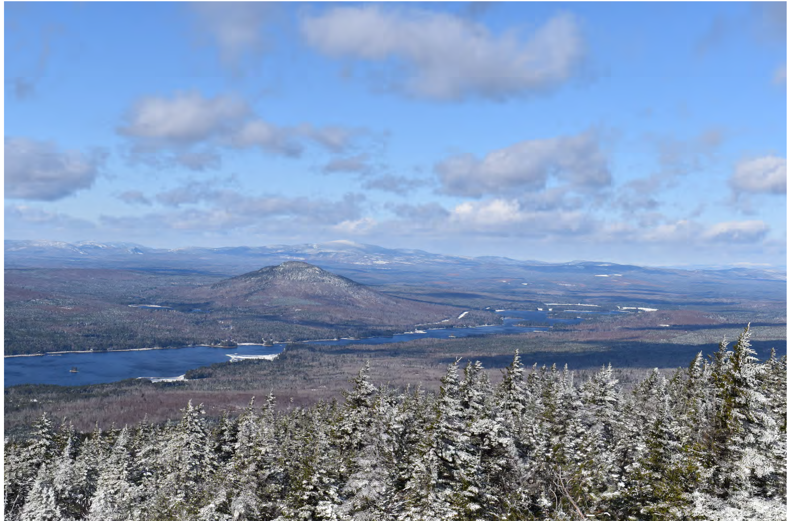
Existing Conditions: Normal view looking northwest from the summit of Bald Mountain in Bald Mountain Twp T2 R3 toward the existing 115 kV transmission line. Mosquito Mountain is visible in the center of the image.
