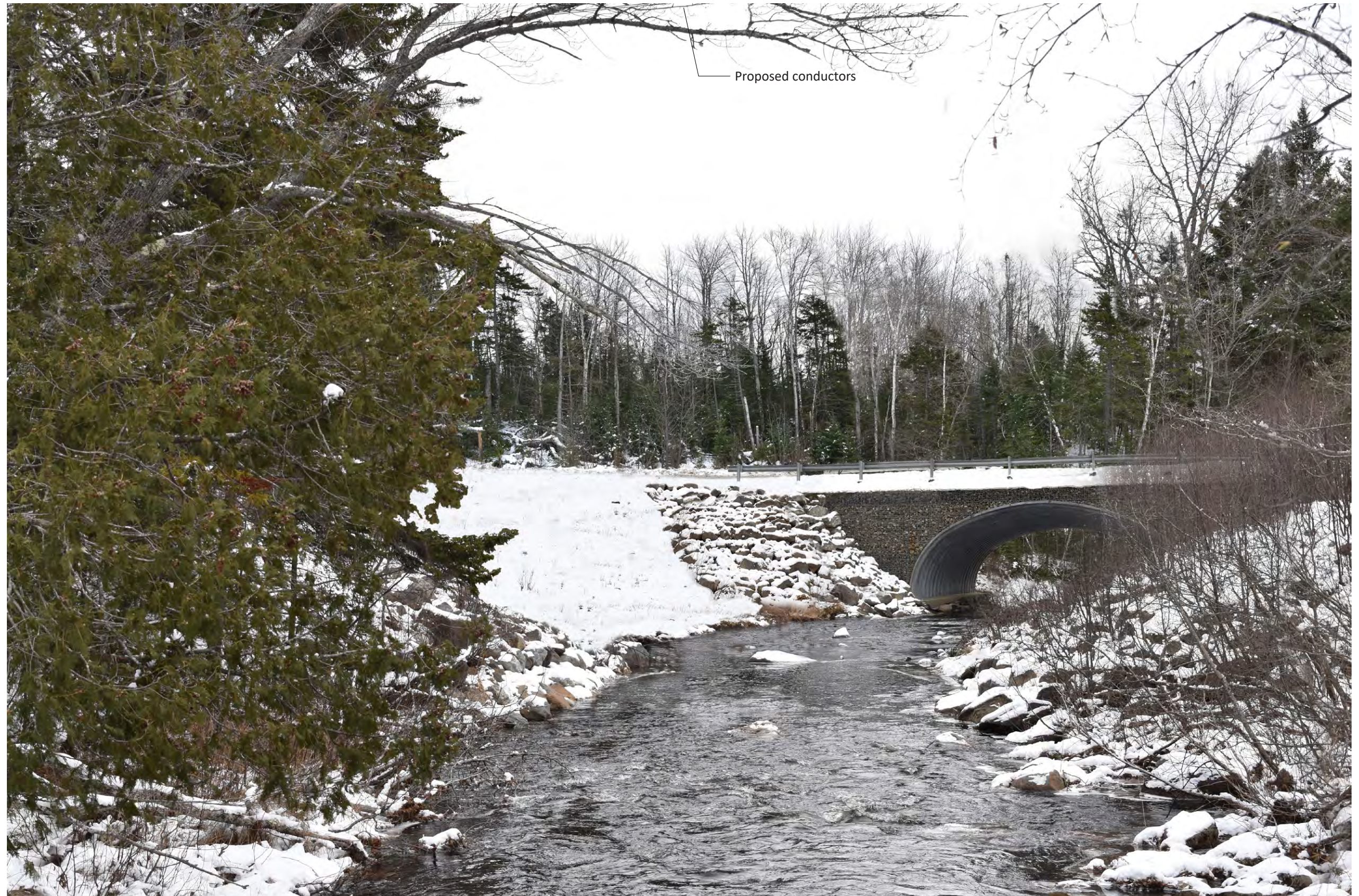
Proposed Conditions: Normal view looking east on the ITS 87 bridge over Cold Stream toward the Capital Road bridge, and the proposed HVDC transmission line. Conductors will be visible crossing above Cold Stream at a distance of 250 feet from this viewpoint.
