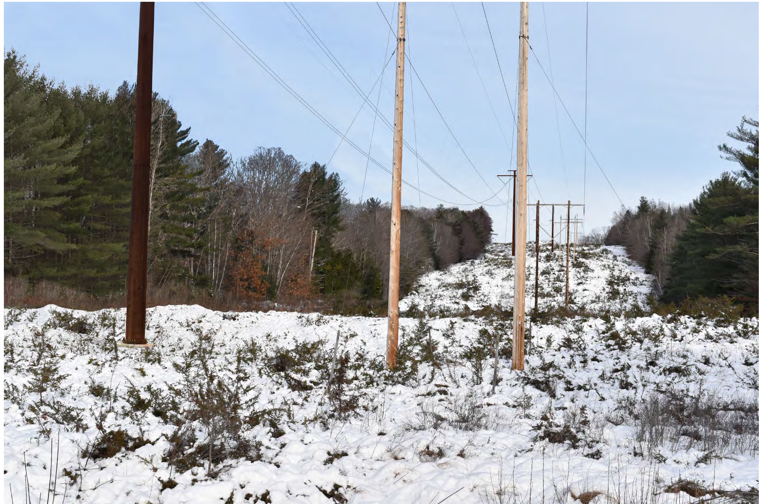
Proposed Conditions: Normal view looking northeast toward the proposed co-located HVDC transmission line from Route 201 in Moscow. The existing 225 ft wide corridor clearing will be widened by 75 ft on the western side (left of corridor in image) to accommodate the proposed HVDC transmission line. Three structures will be visible from this viewpoint.
