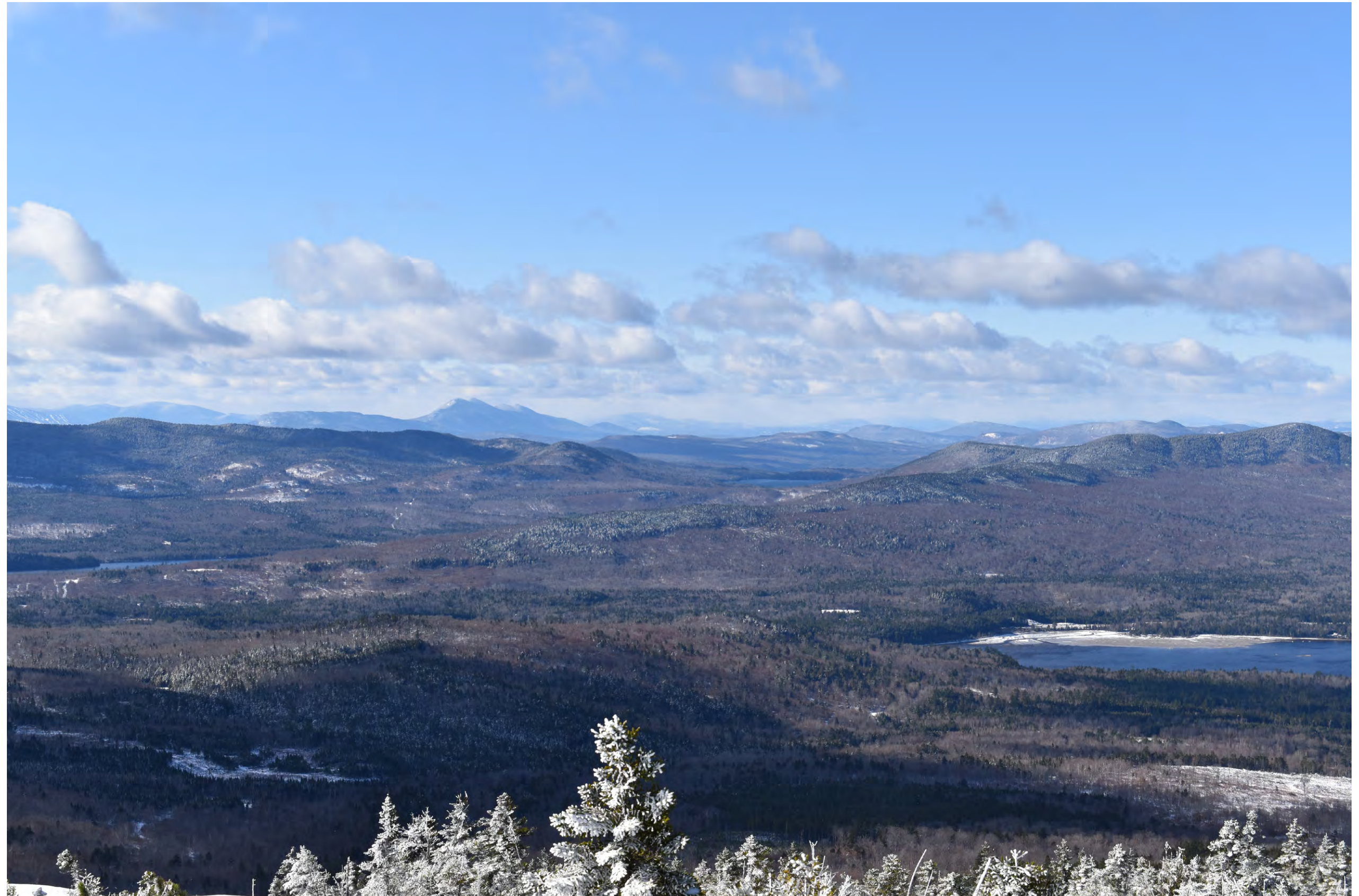
Existing Conditions: Normal view looking west toward the existing 115 kV transmission line from the summit of Bald Mountain, in Bald Mountain Twp T2 R3. Pleasant Pond Mountain is visible on the right side of the image.
