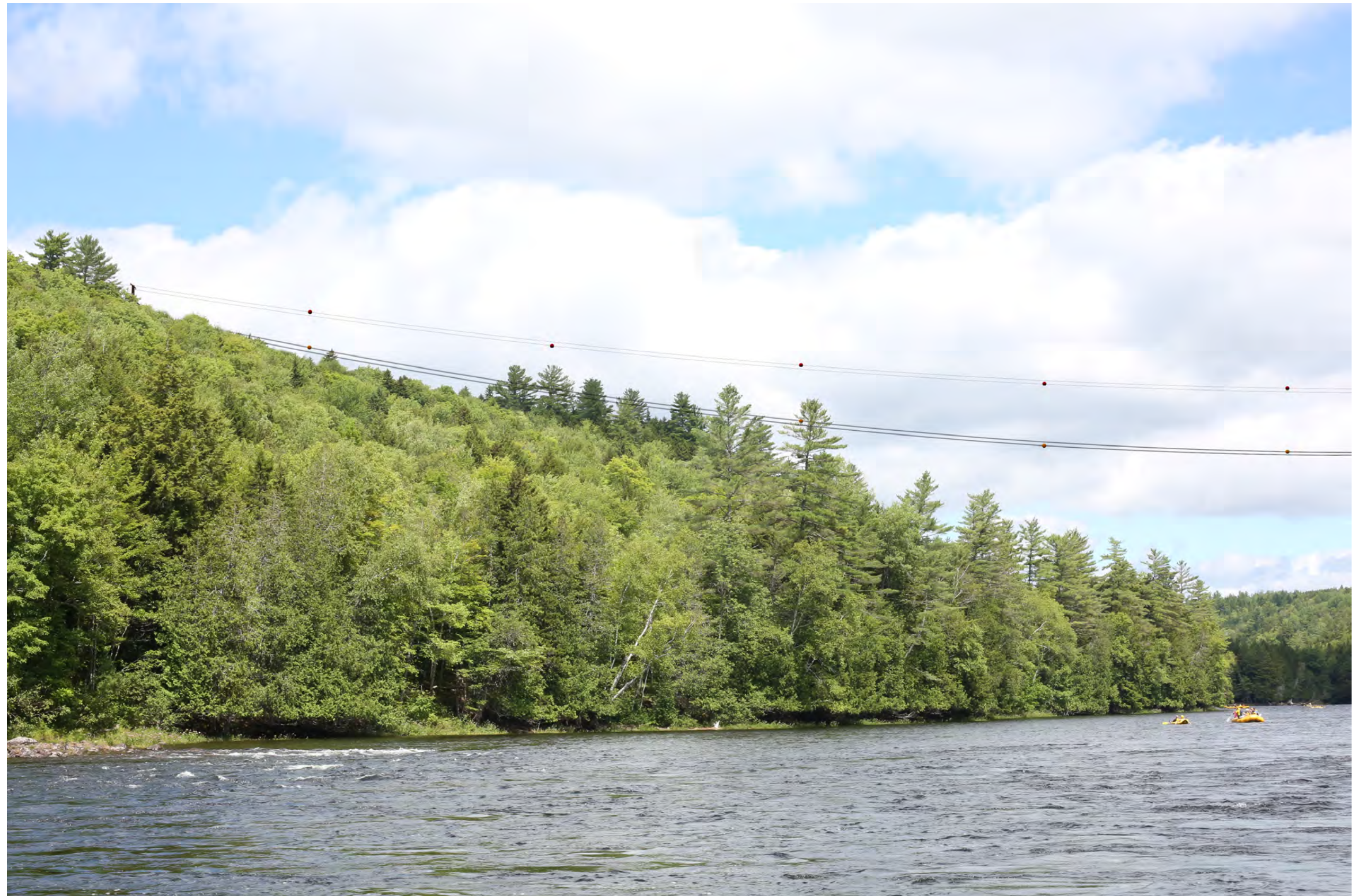
Proposed Conditions: Normal view looking northeast from near the picnic area on the Kennebec River 1,400' +/- south of the proposed HVDC transmission line crossing. The top of one structure will be visible from this viewpoint at a distance of 1,530'. The lowest point of the conductors would be approximately 200' above the water level. Approximately eighteen marker balls will be placed on the shield wires and conductors above the Kennebec Gorge.
