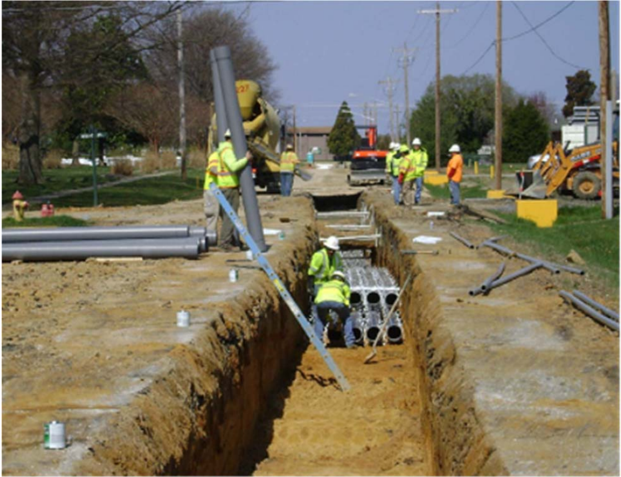
Figure 1 - Duct Bank Excavation
