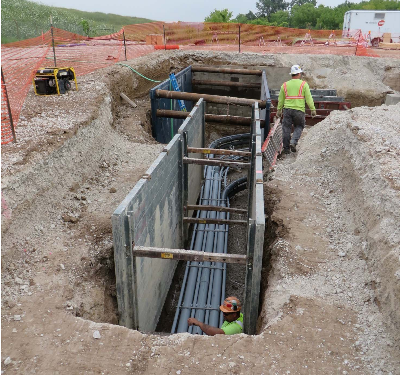
Figure 2- Duct Bank Excavation
