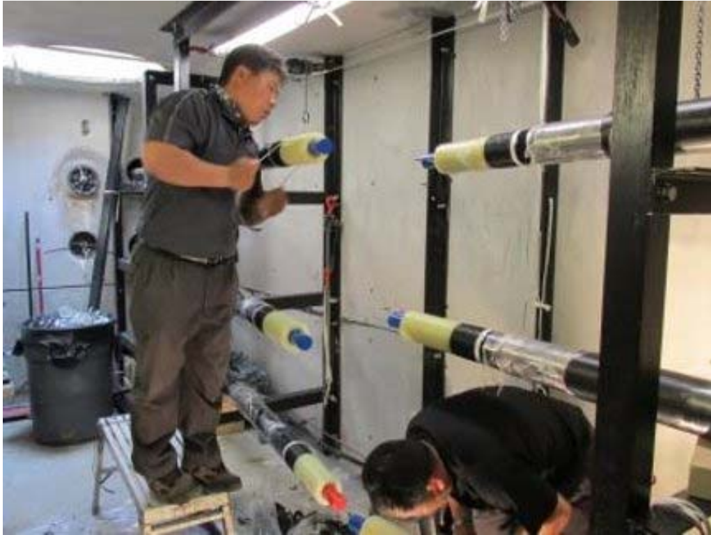
Figure 13 - Preparing Cable for Jointing
