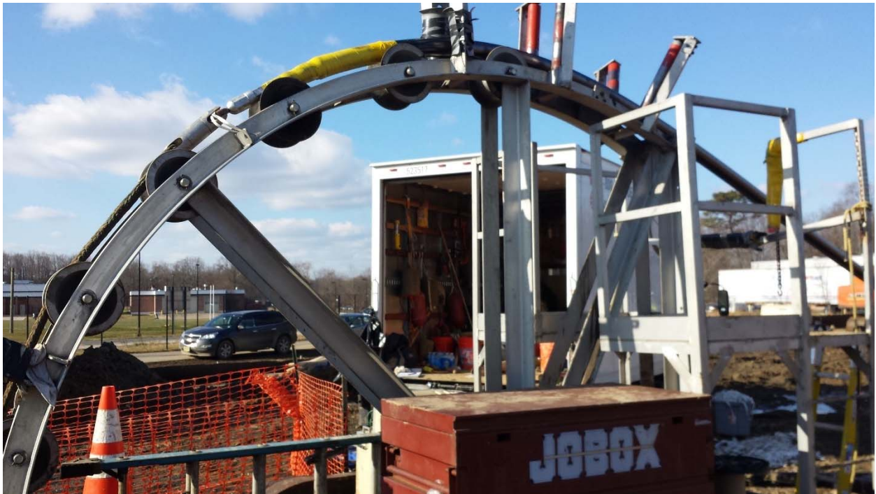
Figure 12- Cable Pulling over Bullwheel
