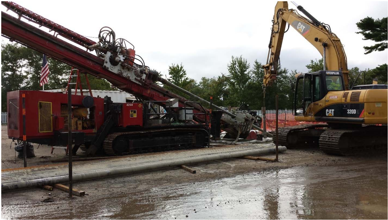
Figure 7 - HDD Drill Rig
