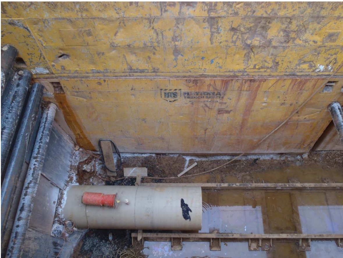
Figure 8 - Pipe Jacking Shaft
