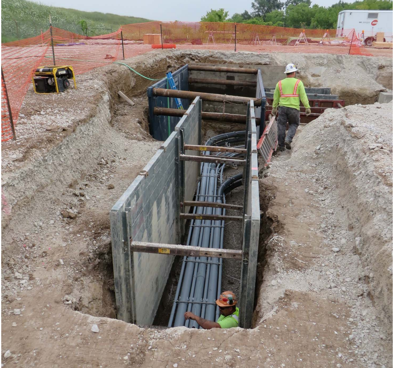
Figure 2- Duct Bank Excavation
