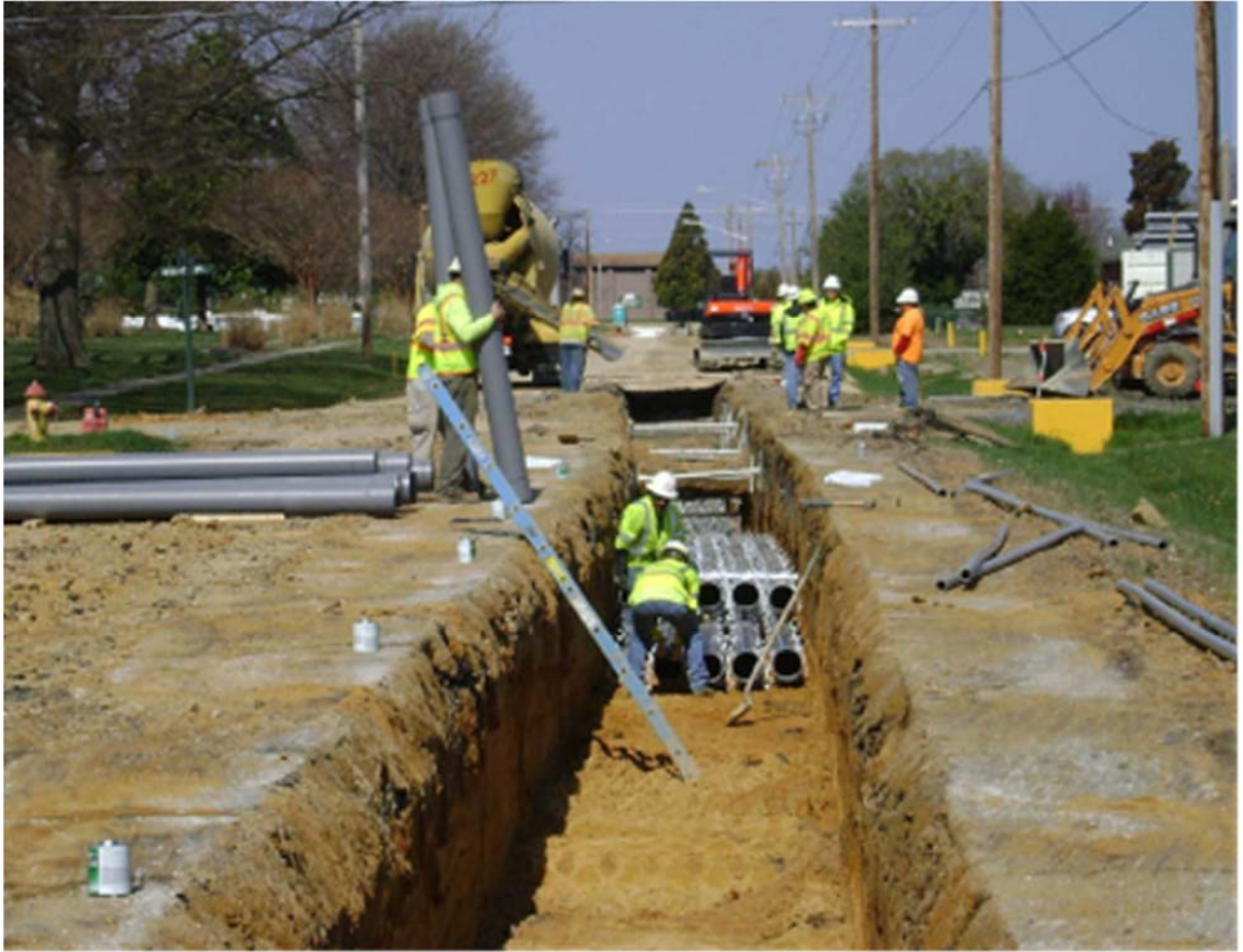
Figure 1 - Duct Bank Excavation
