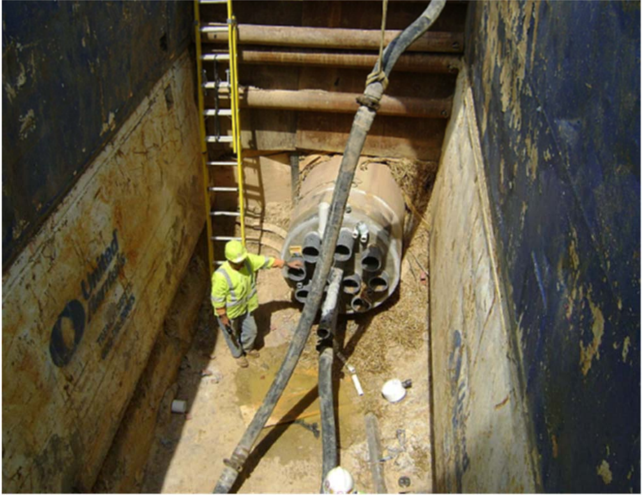
Figure 9- Pipe-Jacking Shaft
