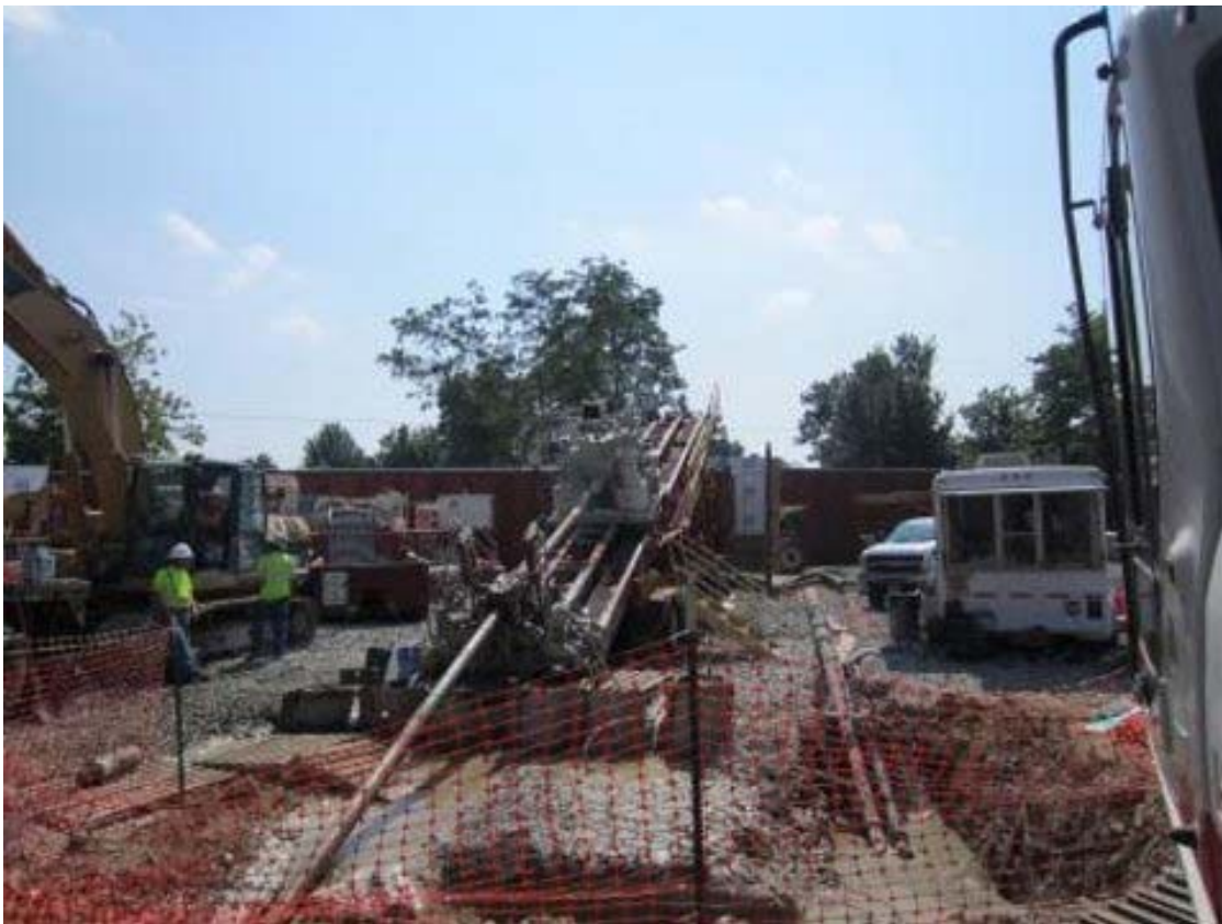
Figure 6 - Horizontal Directional Drill Rig
