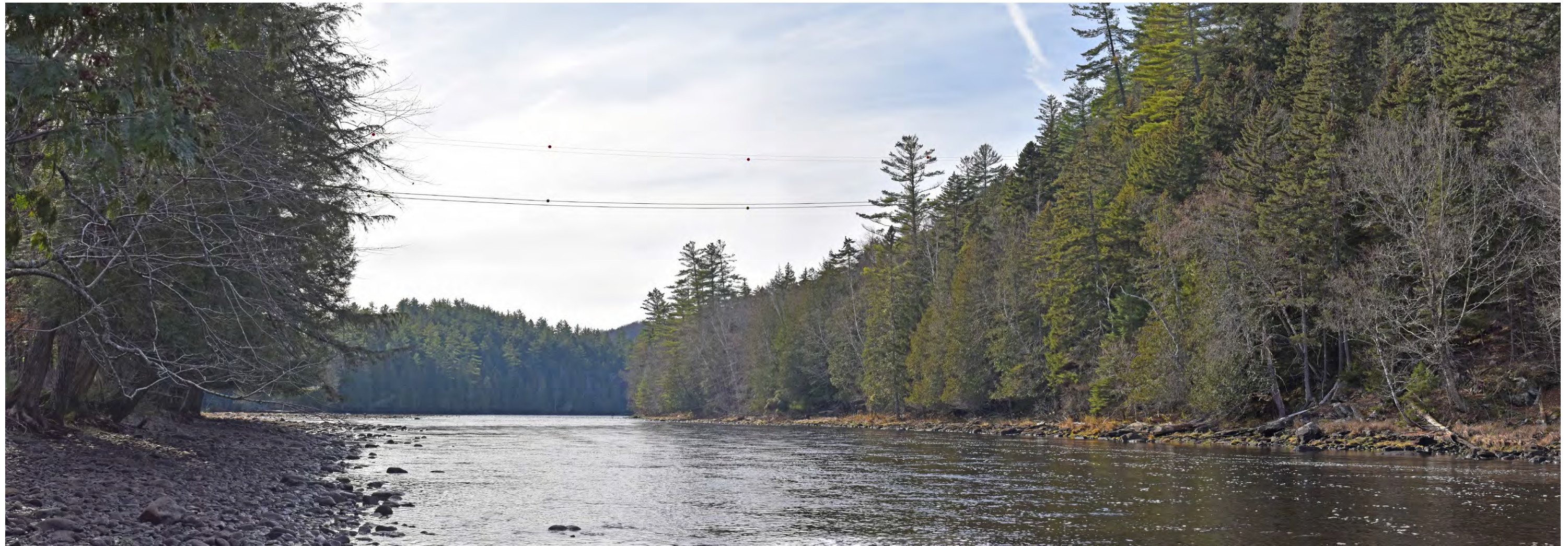
Proposed Conditions: Panoramic view looking southwest from a point 1,150' +/- north of the proposed HVDC transmission line crossing of the Kennebec River, north of a picnic area. The closest structure, screened by vegetation in this view, is 1,250' +/- to the southwest. Conductors, approximately 200' above the river, will be visible to recreational boaters for approximately 1,600' approaching the crossing. Marker balls will be visible on the shield wires and conductors.
