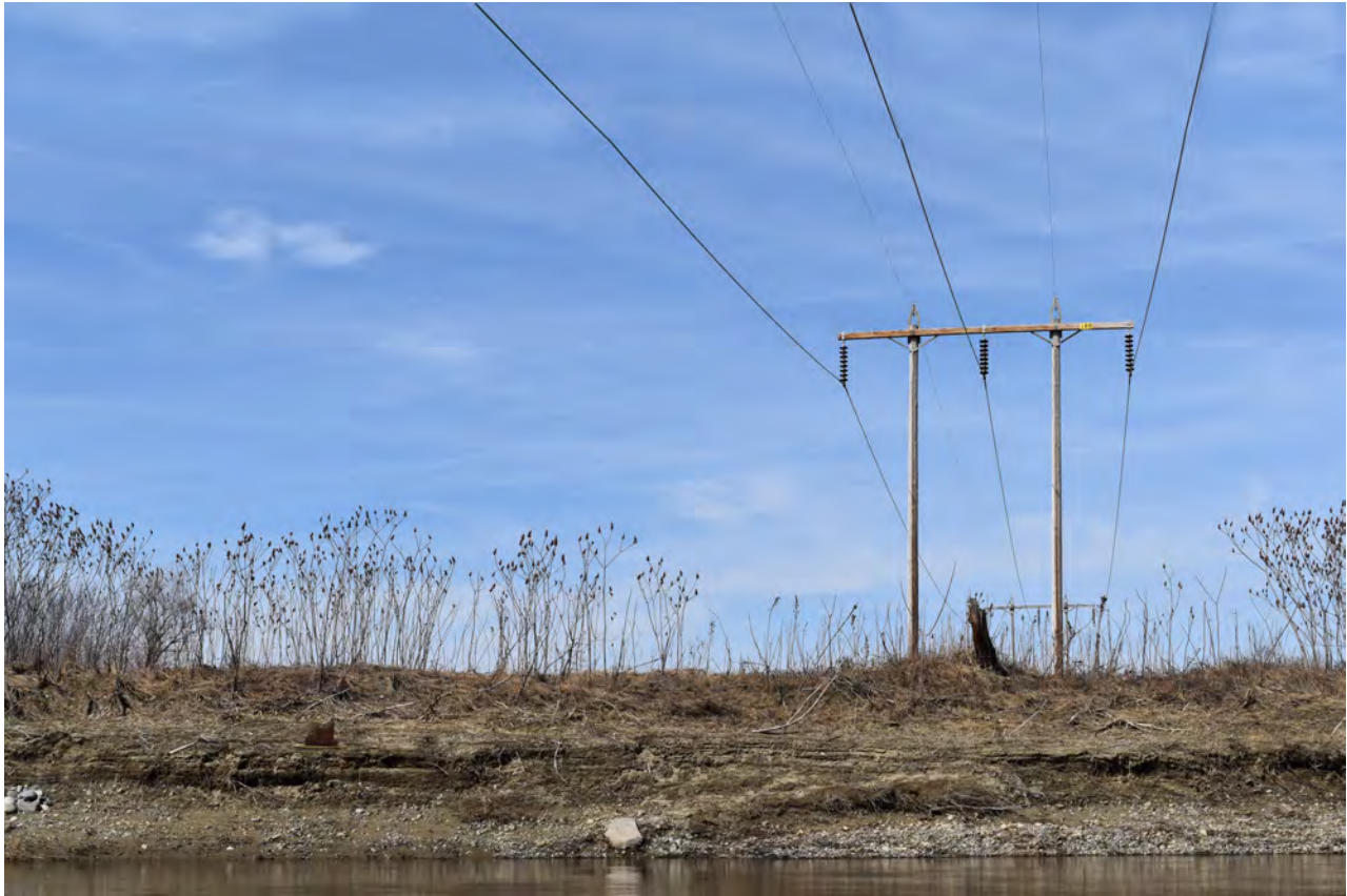
Existing conditions view looking north from Sandy River in Farmington. The closest existing 115kV transmission line structure is approximately 100 feet from the edge of the river.
