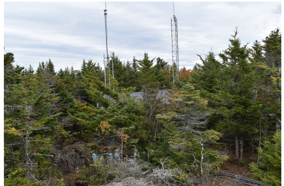
Photograph 15: View looking north toward a building with communication towers on the summit of Moxie Mountain in Caratunk.
