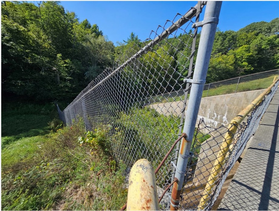
Photo 7 – West Side Downstream Wing Wall
