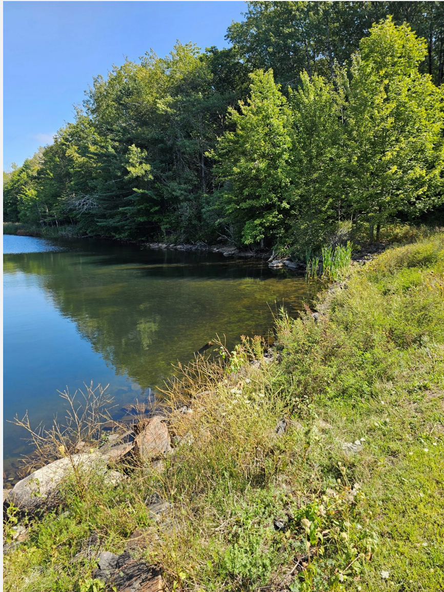
Photo 2 – Earthen Dam Upstream Face East Side
