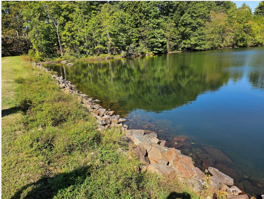
Photo 1 – Earthen Dam Upstream Face West Side
