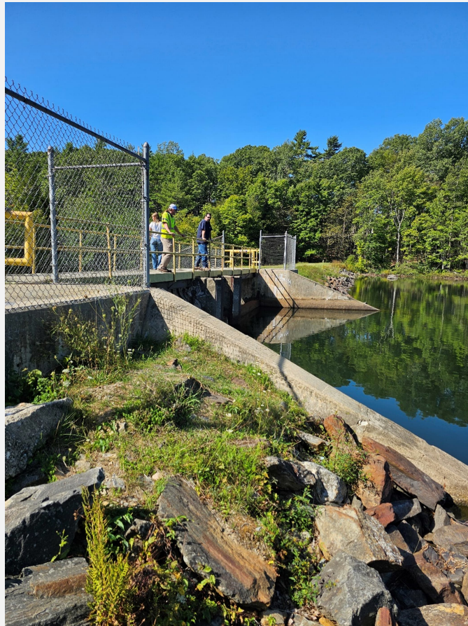
Photo 10 – Upstream Wing Walls and Bridge
