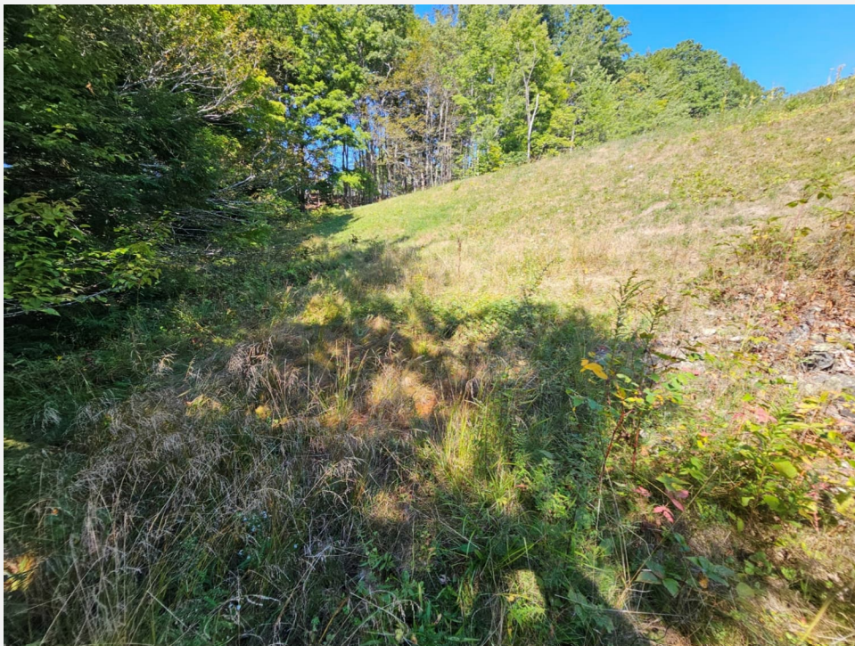
Photo 4 – Earthen Dam Downstream Face East Side
