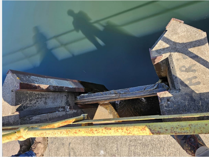
Photo 8 – Downstream Spillways and Gate
