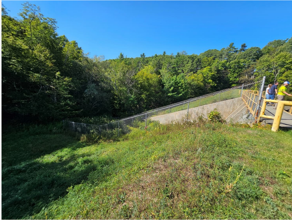
Photo 5 – Earthen Dam Downstream Face East Side
