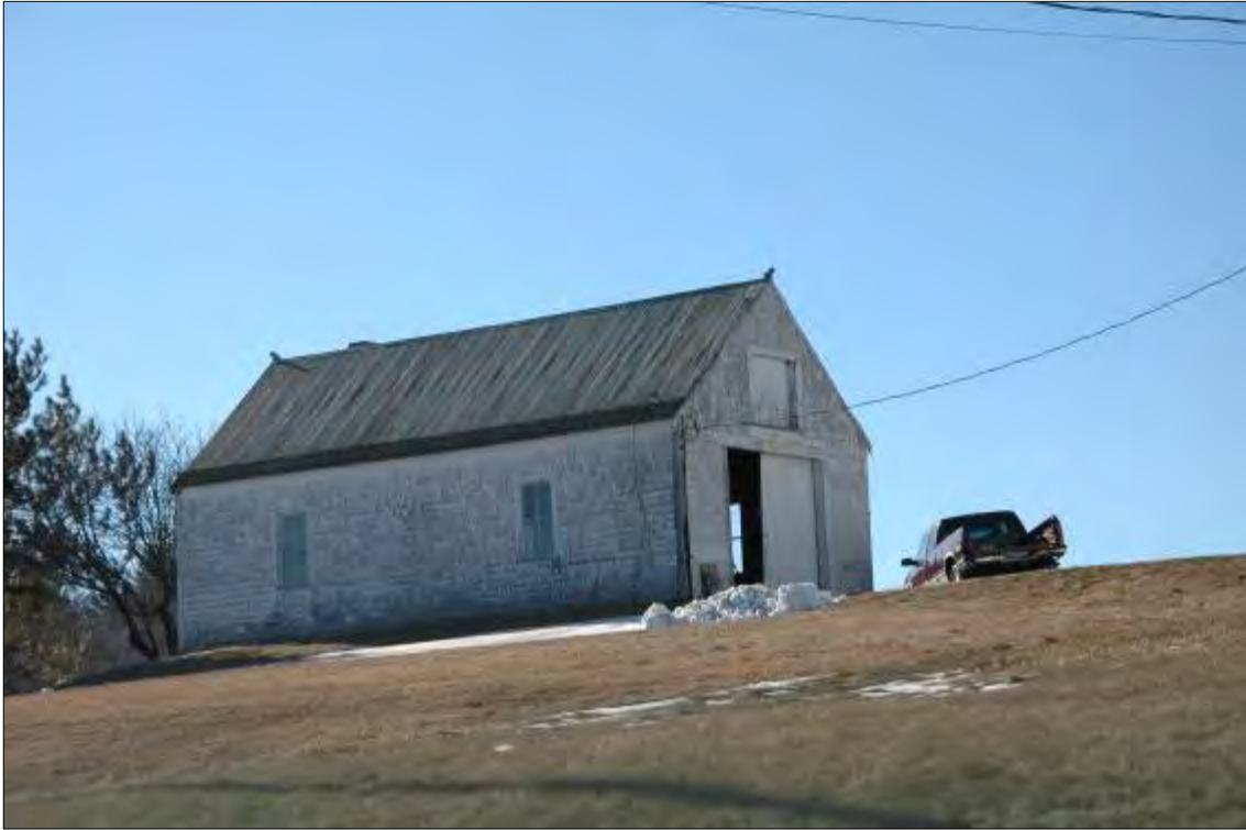
Photograph 9 Workshop Brighton Road/County Road 154, west side of street, approx. 1580 feet south of the intersection with Main Street/County Road 154 (Survey Map No. 68).
