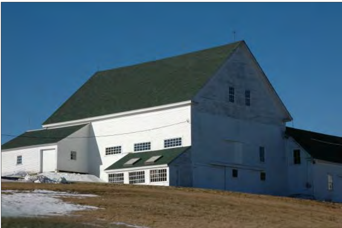
Photograph 8 Barn, Brighton Road/County Road 154, west side of street, approx. 1580 feet south of the Photograph with Main Street/County Road 154 (Survey Map No. 67).
