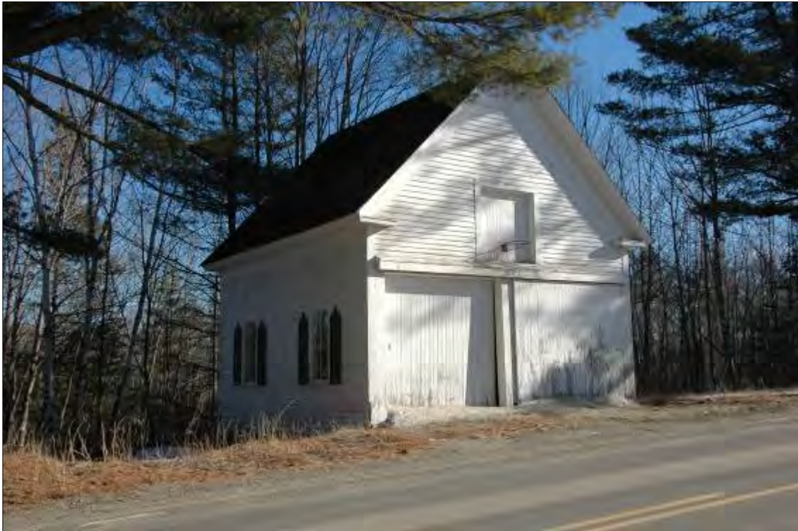
Photograph 11 Garage, Brighton Road/County Road 154, west side of street, approx. 1580 feet south of the intersection with Main Street/County Road 154 (Survey Map No. 70).
