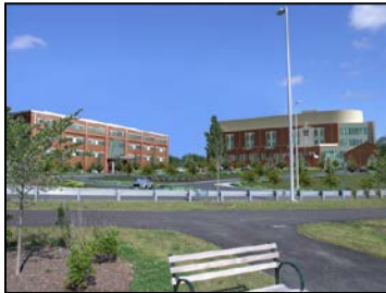
Mercy Hospital Relocation
